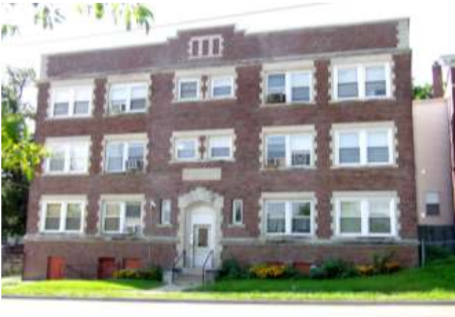
Front Façade – 812 Forest Ave 6 units, currently occupied
