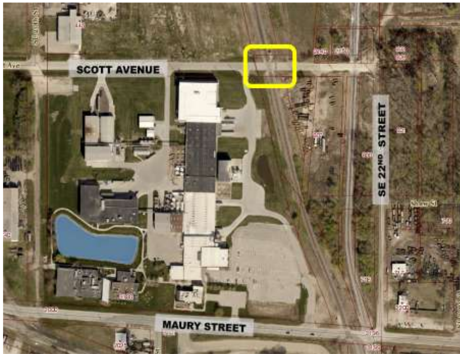
SCOTT AVENUE CROSSING
