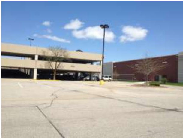
a. View from parking lot fronting Douglas Avenue looking north at parking ramp proposed for demolition.
