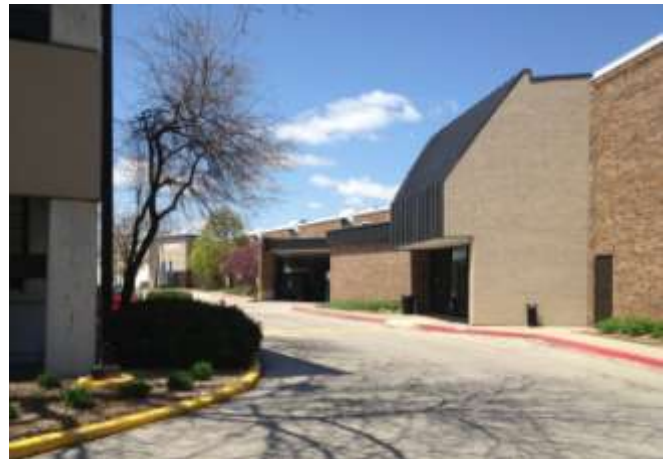
b. View of mall's south entrance area from interior drive. To the left is the ramp to be demolished.
