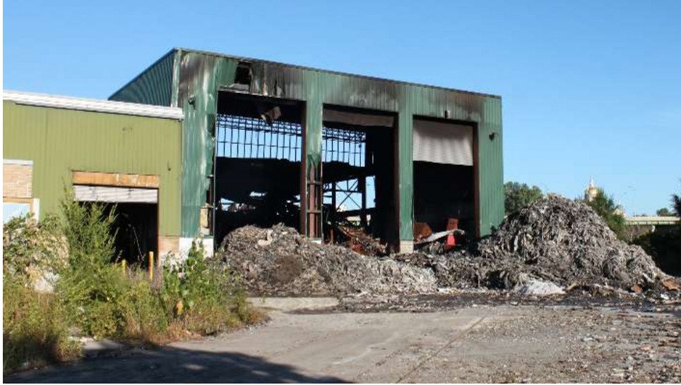
1422 Scott Avenue After Fire – September 2013
