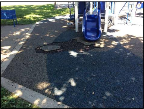
• These large areas are too large to patch and with the failing binder it was determined that the only solution is to completely remove the existing playground surfacing and replace it with an upgraded new poured-in-place rubber playground surface. The new system, which will still be two (2) layers, will have a much-improved Aliphatic Urethane binder.
