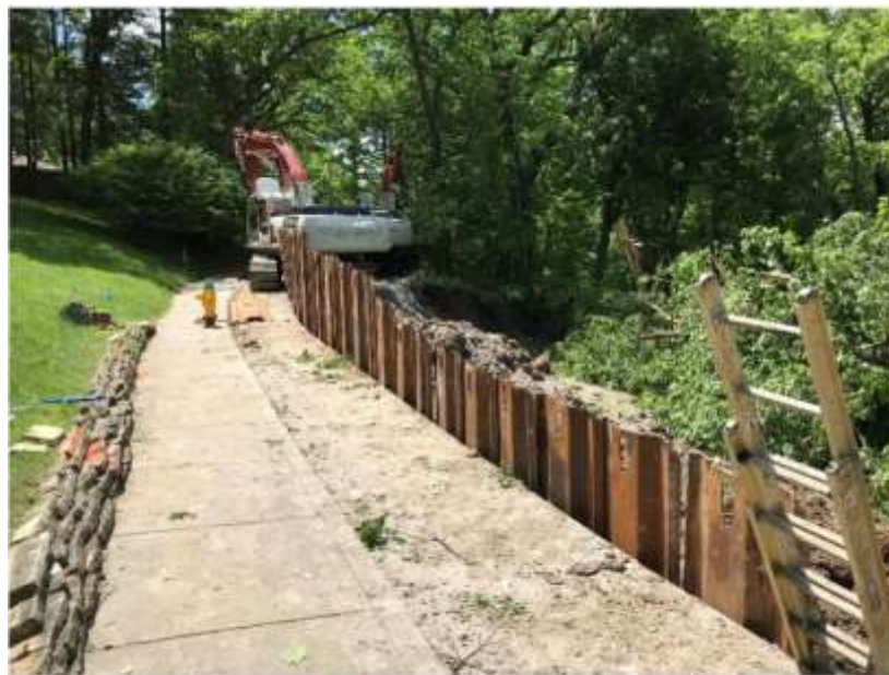
Image 2: View looking SW after sheet pile installation.
