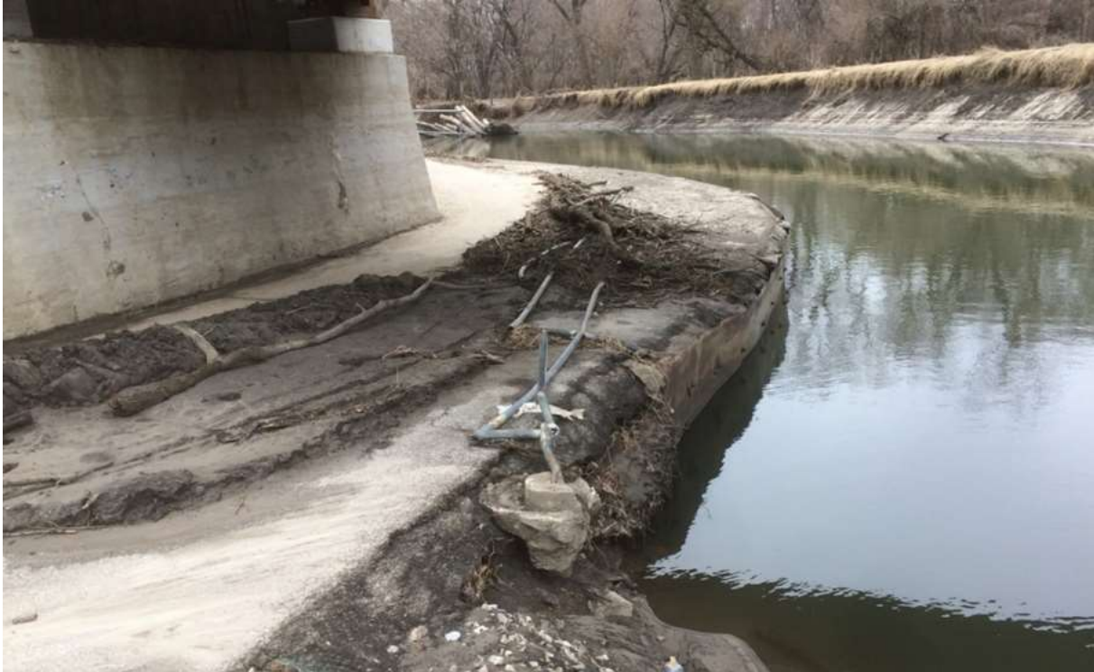
Photo of Underpass Damage Following 2019 Flood Event
