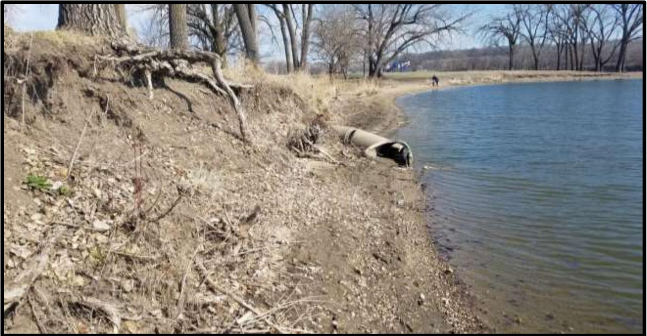
Photo above: North-centrally located 6-foot tall eroded lake shoreline and damaged storm sewer.
