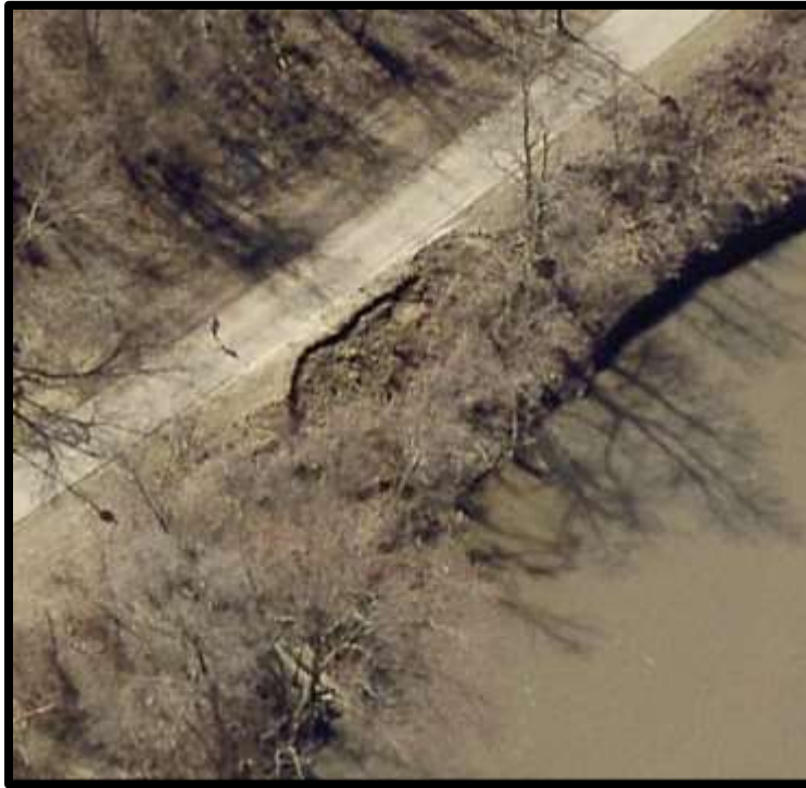
Photo Above: Oblique Aerial of Erosion
