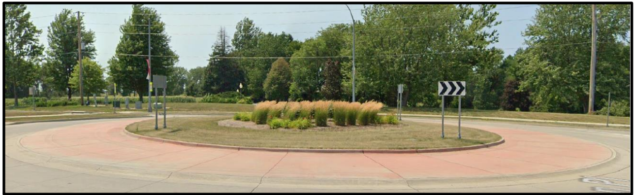
Above Graphic: Example (Precedent) Roundabout at University Avenue and Collaboration Place, Ames, Iowa (SE 36th Street/E. Army Post Road Roundabout will look similar)
