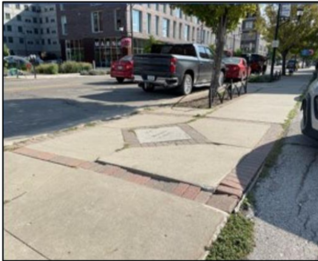
Above Left Image: Existing settled brick banding, sidewalk and county plaque.
