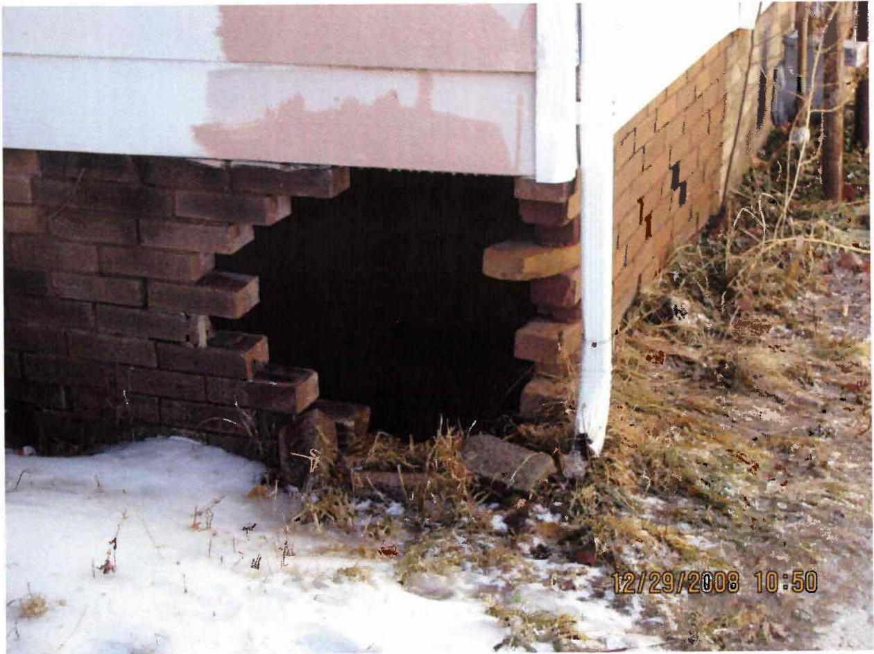
1702 Forest North Basement Wall.
