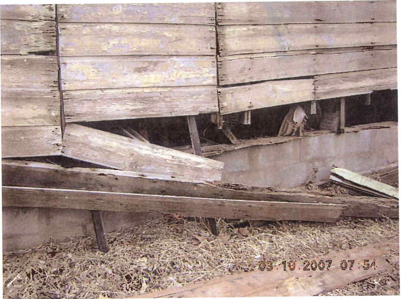
1427 10 TH EAST GARAGE WALL.
