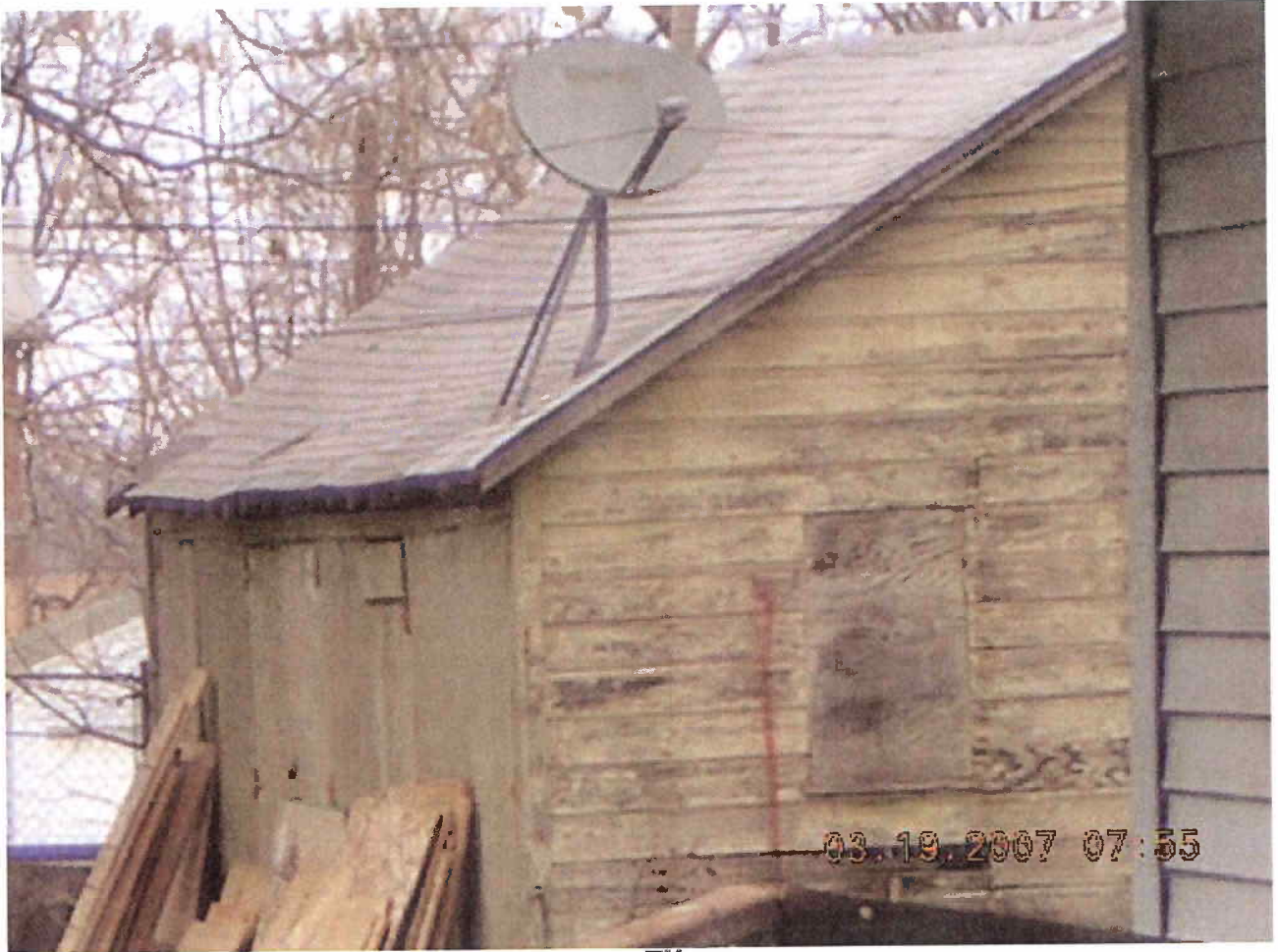
1427 10 TH WEST VIEW OF GARAGE ROOF.
