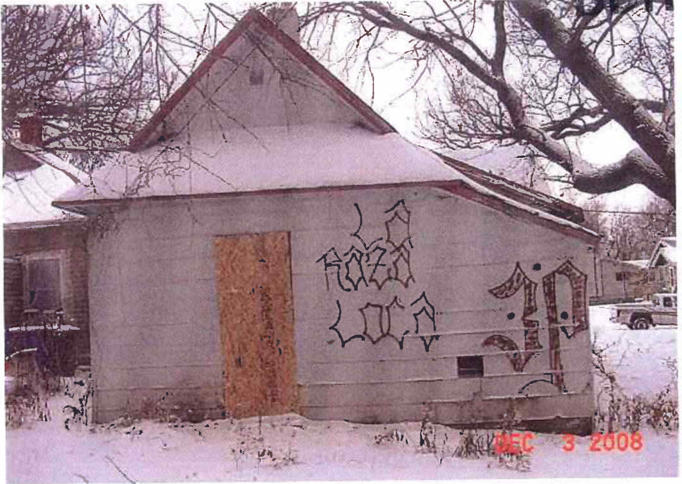
2110 MEEK AVENUE REAR (south)
