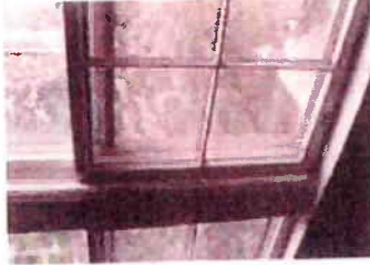
Not Recommended: [31-32] Ill-fitting exterior aluminum storm windows viewed from both inside and outside are clearly not energy efficient.
