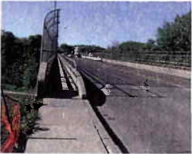
6th Avenue Bridge Spring 2012 Before rehabilitation
