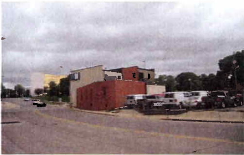
West elevation (terracotta paint on second floor)
