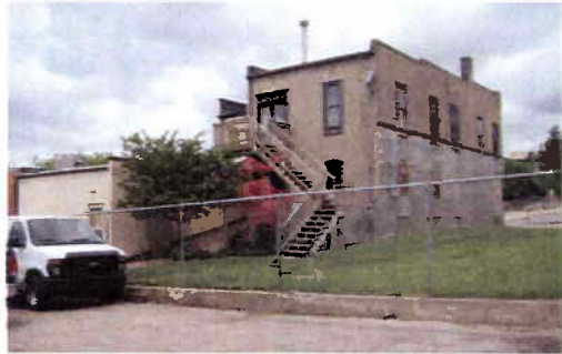
South and east elevations
