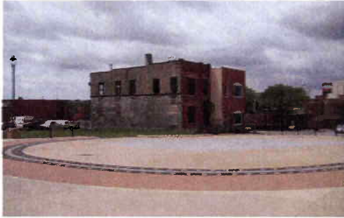
East and north elevations
