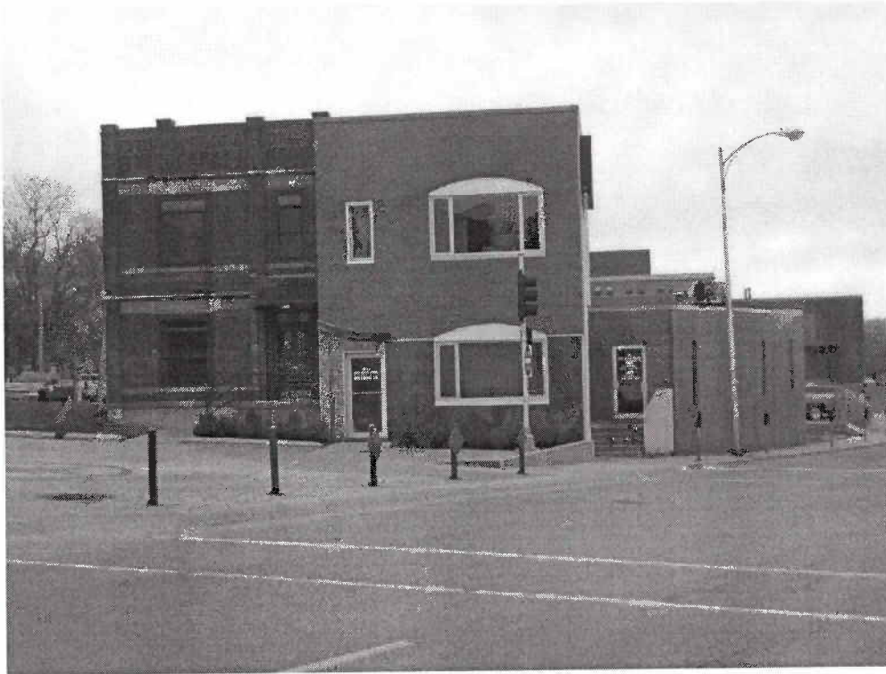
Photo 1: Samuel Green Rowhouse–Norden Hall, 709 E. Locust Street, pictured on left. To the right is 707 E. Locust Street. Photo taken from Pennsylvania Avenue looking southeast. (May 30, 2013)
