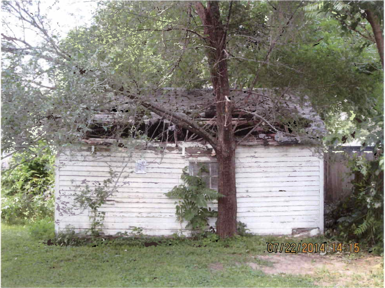
700 E. GRANGER SOUTH SIDE OF GARAGE
