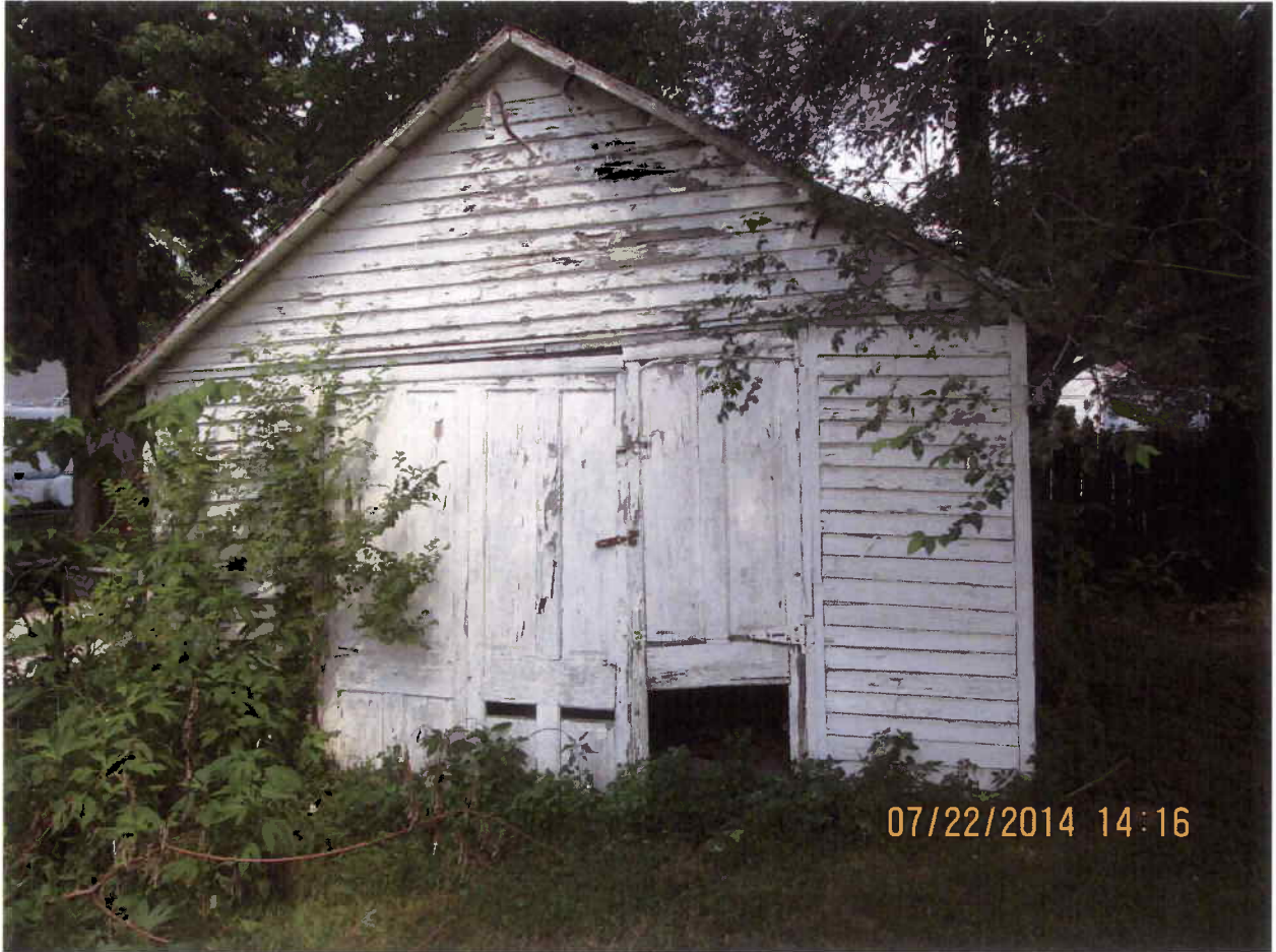
700 E. GRANGER WEST SIDE OF GARAGE
