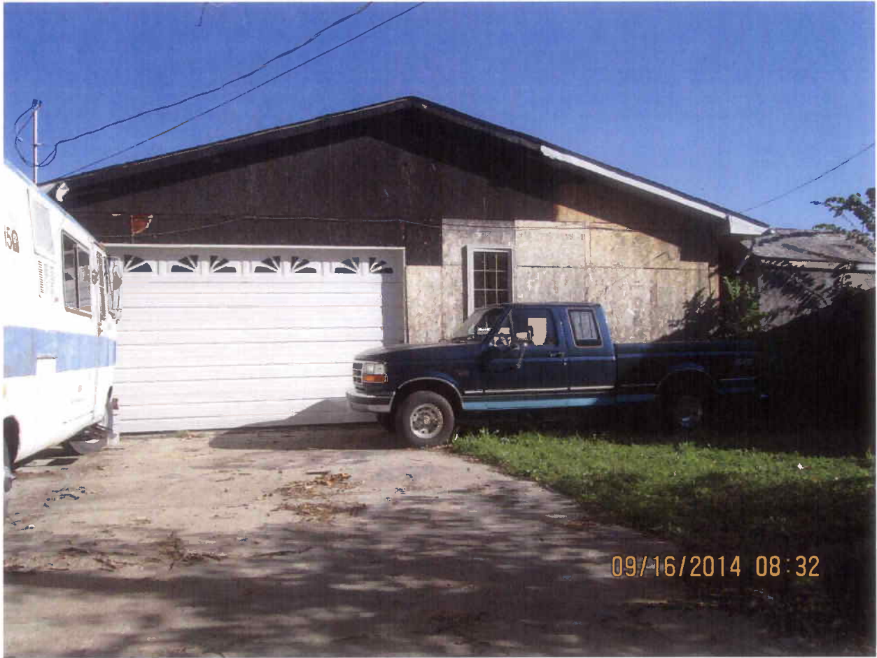
708 Hickman South side of house.
