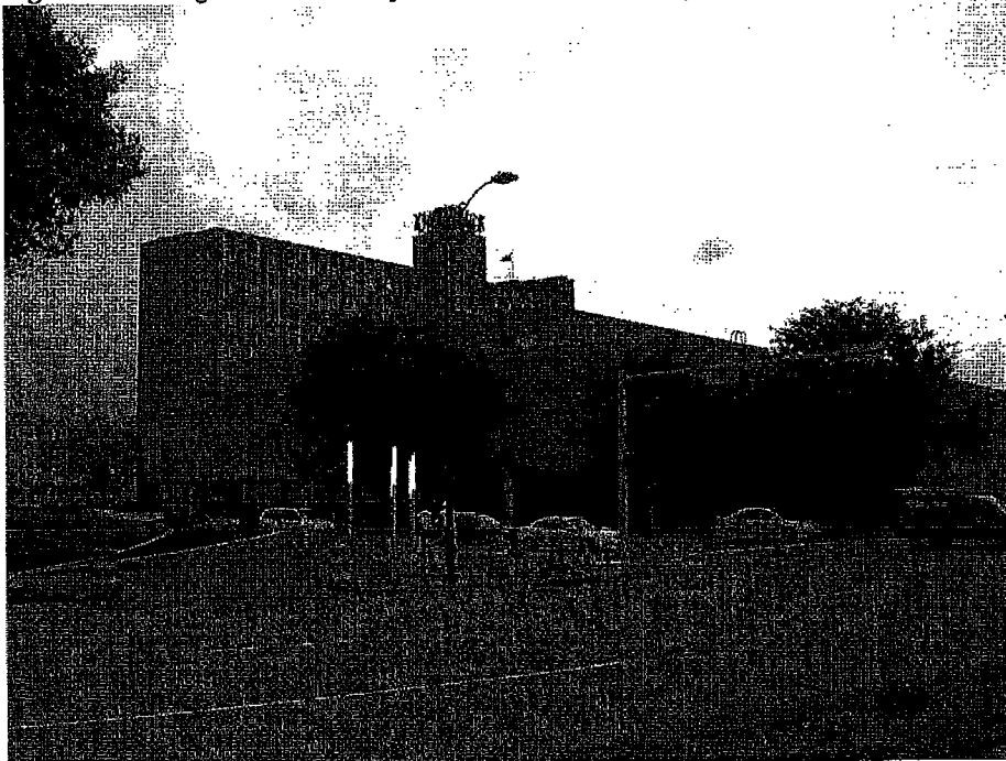
Fig. 14: Looking SE- North Façade, October 2007
