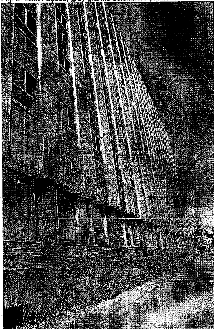
Fig. 5: East Façade, grey granite columns, April 2010
