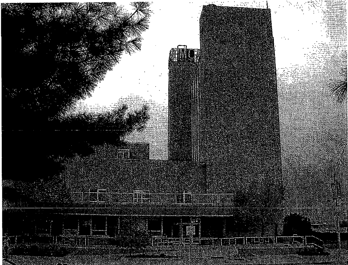
Fig. 8: YMCA, looking N, Locust St. view, central square tower containing elevators, October 2007
