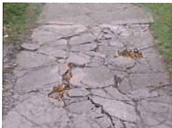
Example of a sidewalk needing replacement
