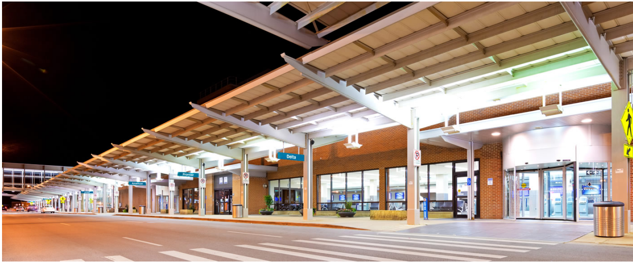
Figure 6.1 DSM MAIN TERMINAL ENTRANCE
