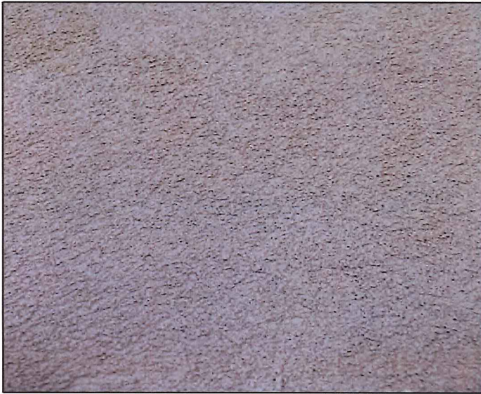
Exterior Insulated Finish System (EIFS)
