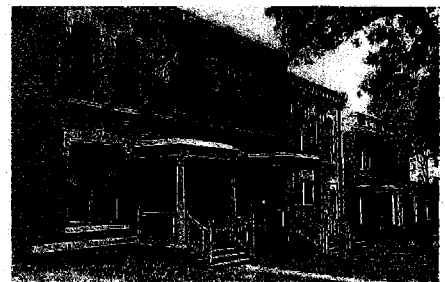
Row House residence, 1880, 733-35 19th Street
