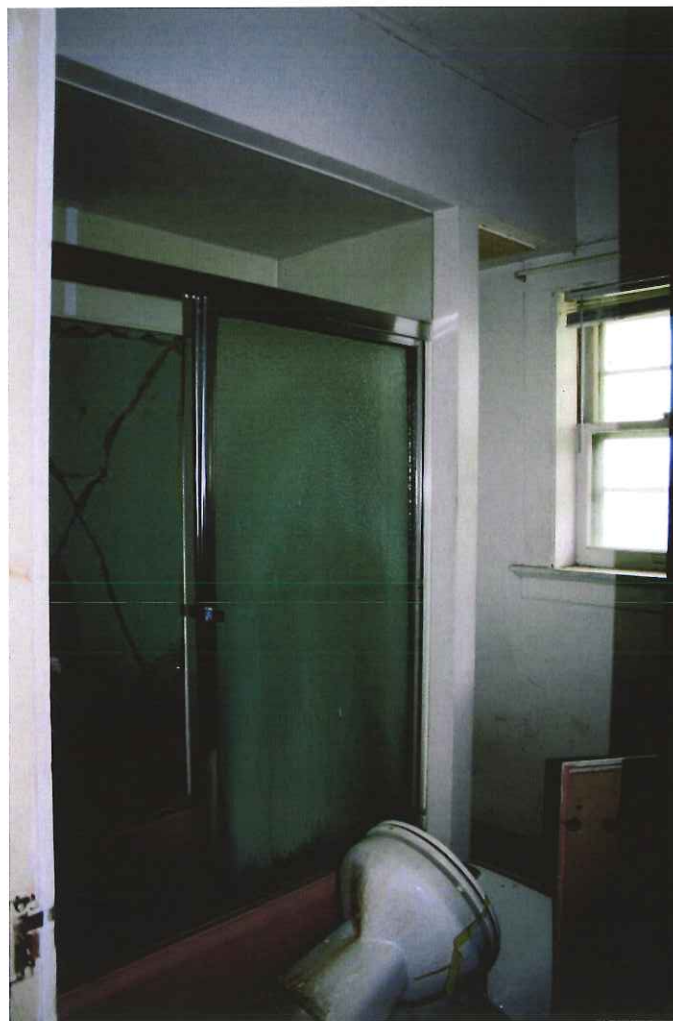
19. Interior 4020: Second floor, bathroom looking SE.
