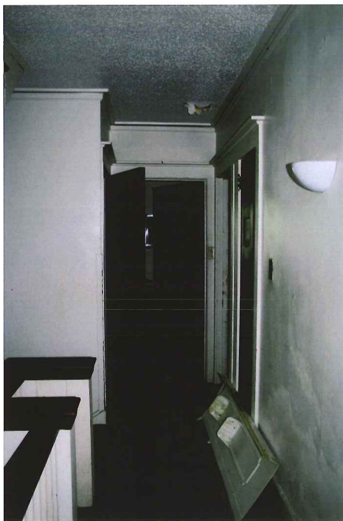
14. Interior 4020: Second floor, hallway, looking south.
