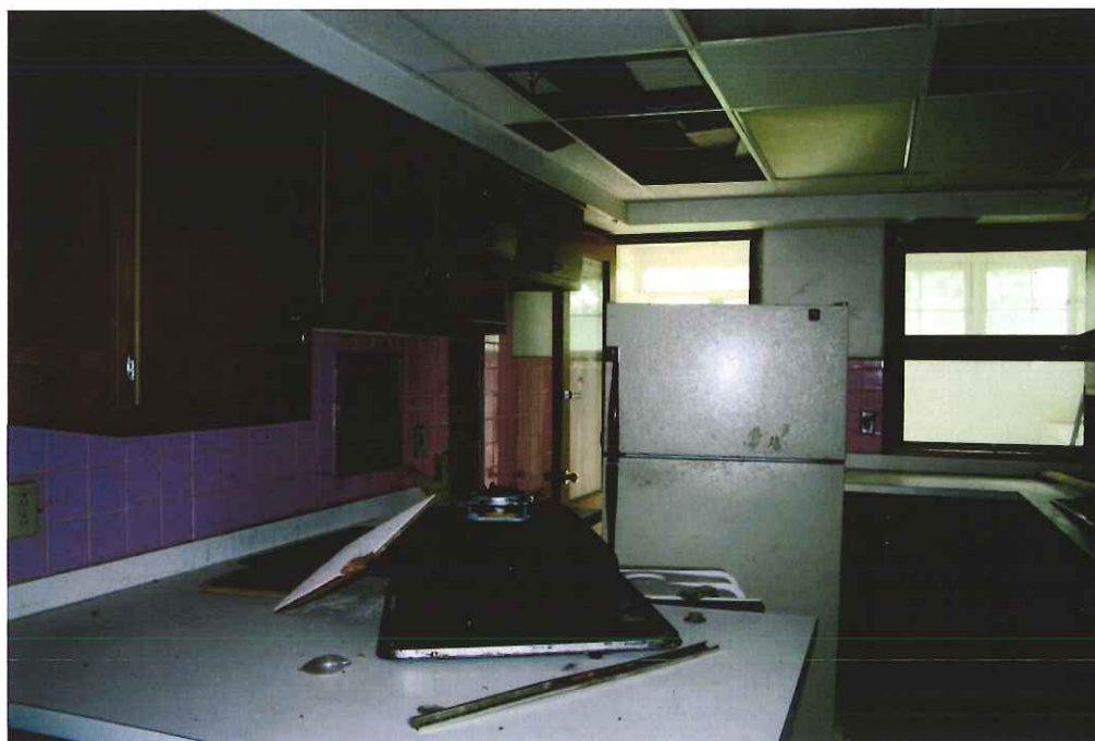
11. Interior 4020: First floor, kitchen looking south toward rear entrance.
