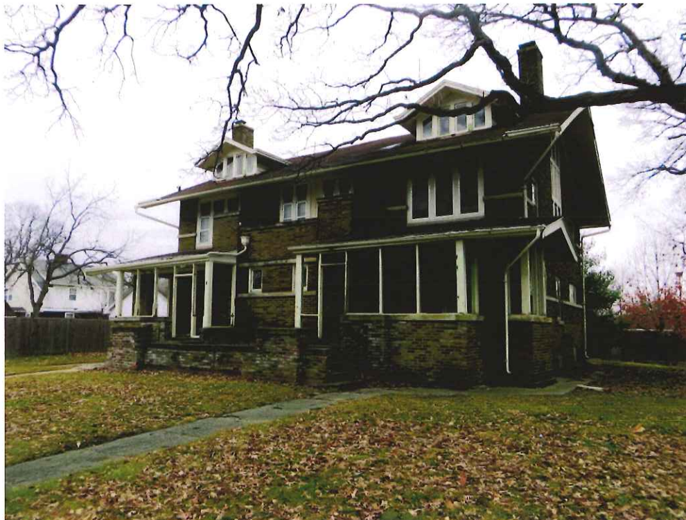
4. Exterior: View of the façade (north) and west elevation, looking SE with 4018 at right.
