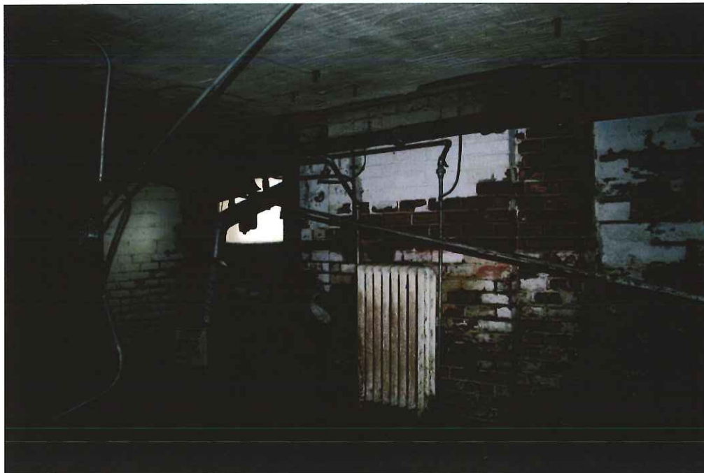
26. Interior 4020: Representative view of the basement.
