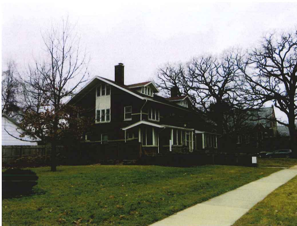
1. Site: View looking SW along Ingersoll Avenue
