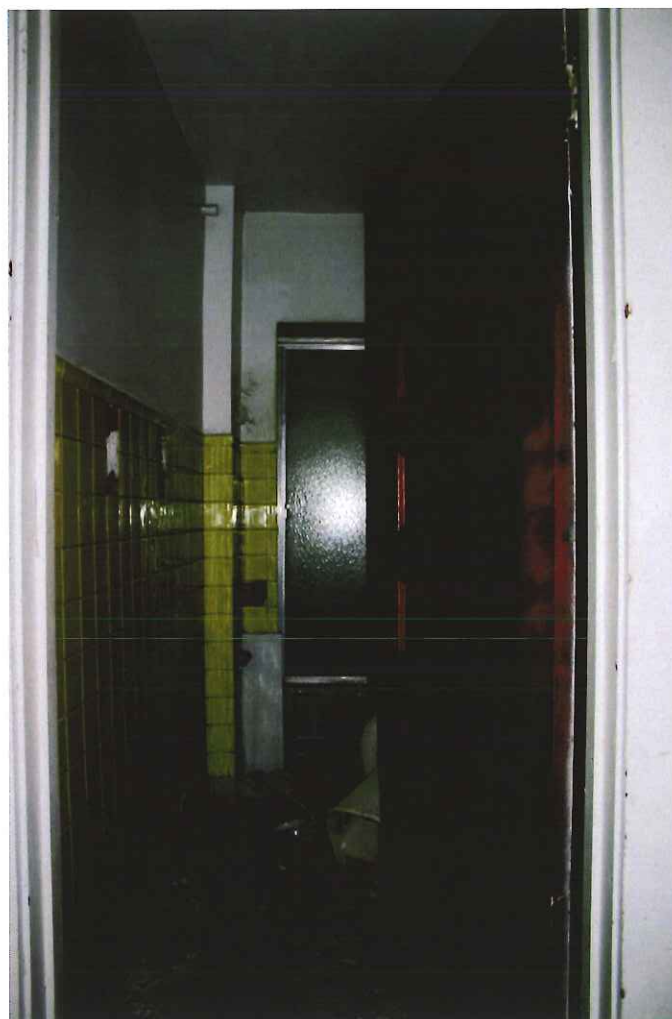
25. Interior 4020: Third floor bathroom, looking south.
