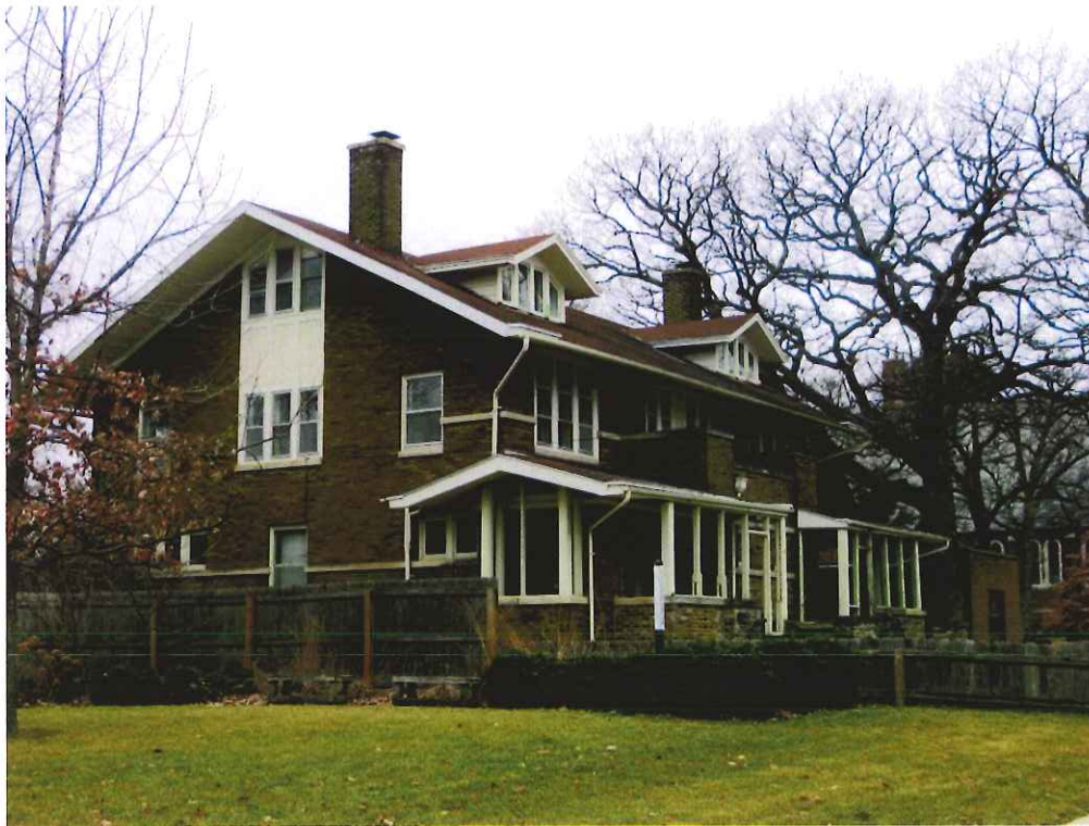
3. Exterior: View of the façade (north) and east elevation, looking SW.
