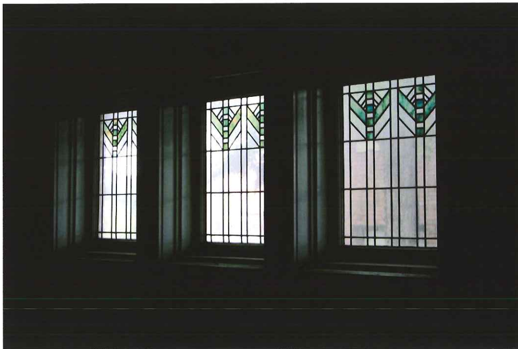
12. Interior 4020: First floor details – stained glass windows, east dining room wall.
