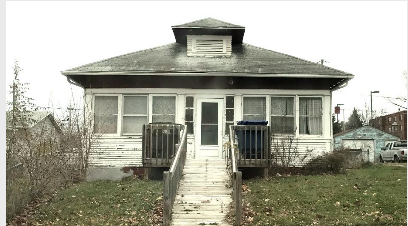
Figure 3. Code enforcement staff currently monitor over 300 vacant properties.
