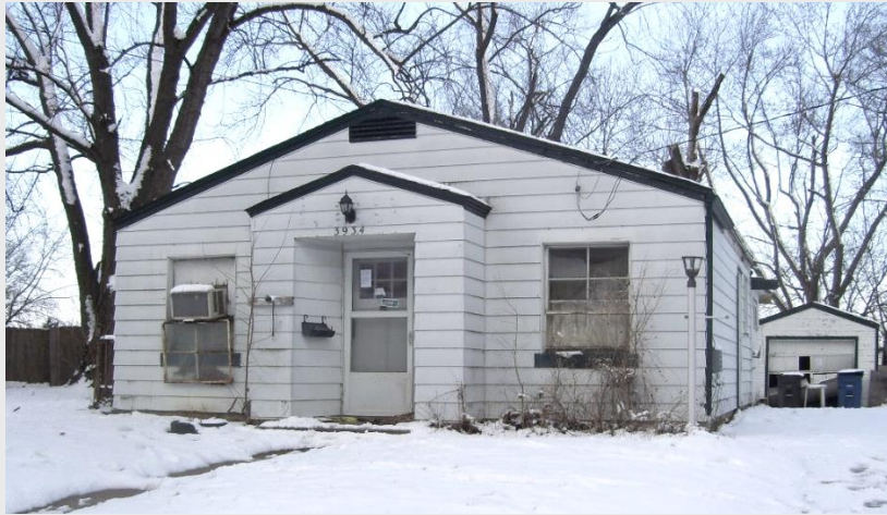
Figure 6. Vacant monitor property. Numerous code enforcement actions since 2002. Previously a rental and contract sale.
