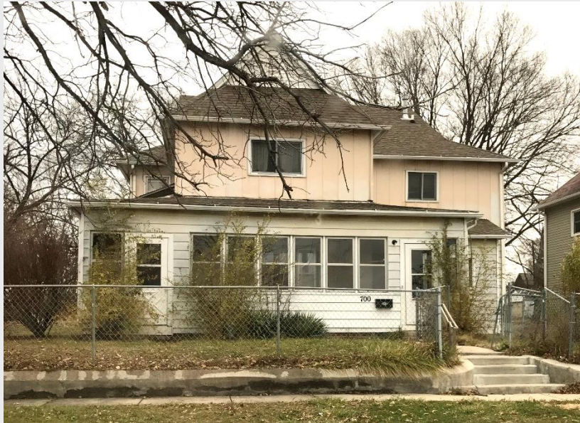
Figure 5. Occupied rental property in below normal condition.
