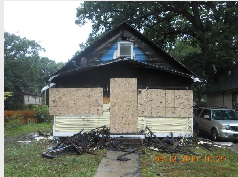
Figure 2. A vacant property becomes fire damaged in 2014.
