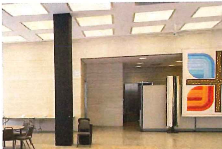
Photo 12. Interior 1st-floor column with potentially original Detroit Graphite as its current finish.
