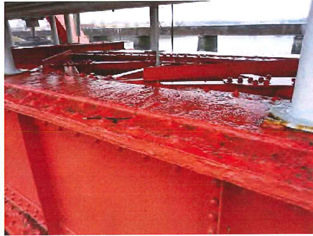
North Girder – Looking Southeast
