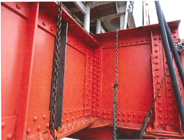
South Girder Connection Pier 2 - Exterior Side
