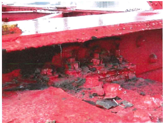
North Girder Connection at Pier 2
