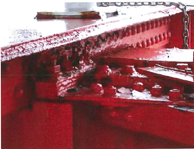
South Girder Connection at Pier 2
