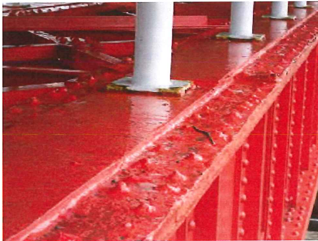
North Girder – Looking West toward Pier 1
