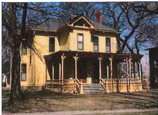
Maish House, 1623 Center St. Listed April 1977
