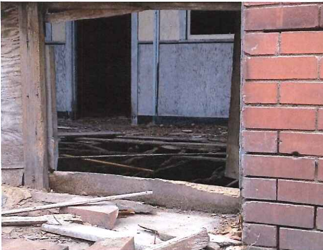
Deteriorated flooring and joists
