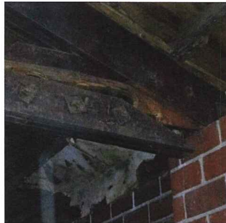
Interior roof truss failure
