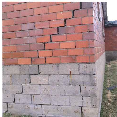
Masonry joint separation from settlement
