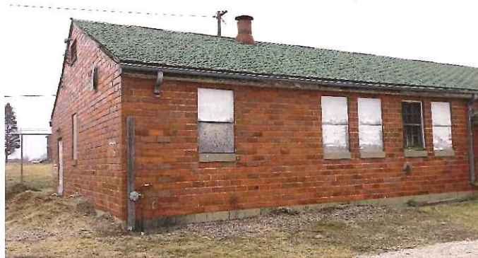
Missing downspout - roof condition
