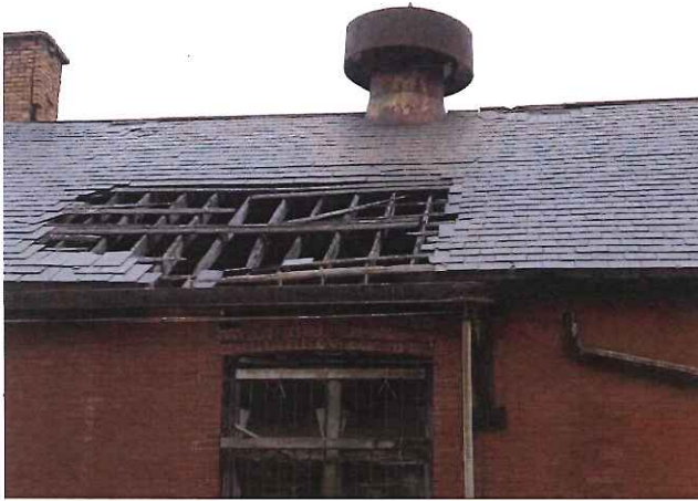
Slate roof and roof structure deterioration
