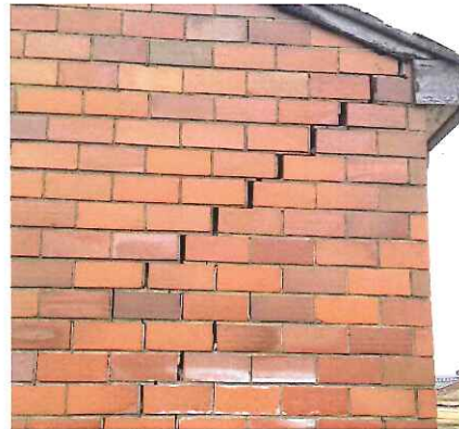
Masonry joint separation
