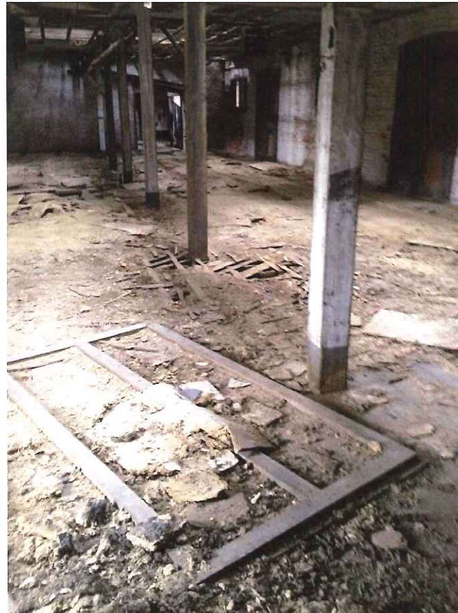
Deteriorated Flooring, Floor Joists and roof structure
