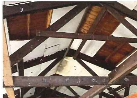
Moisture damage at roof decking
