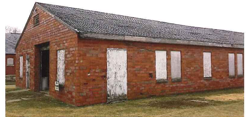
Missing gutters and downspouts - roof sag
