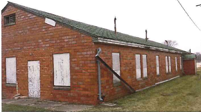
Missing gutter - masonry joint condition
