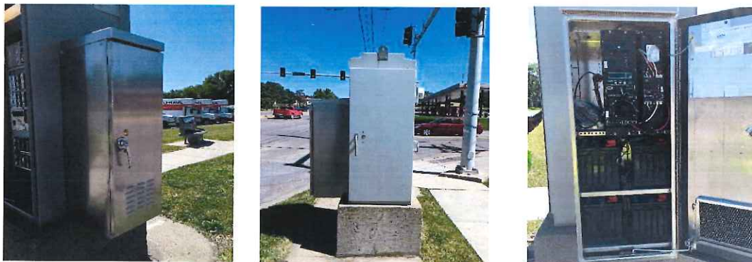
Figure 12 –Battery Backup System
