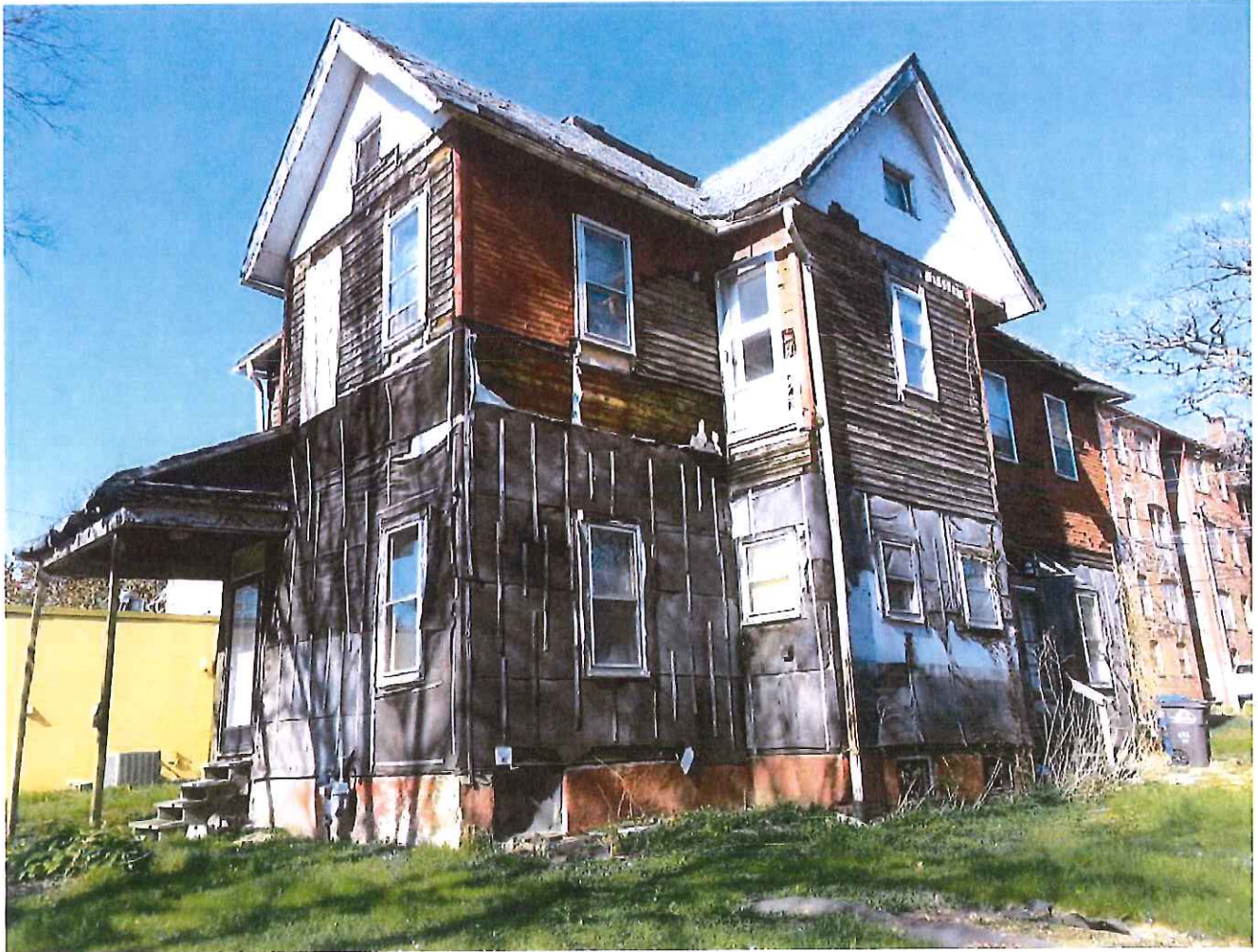
1-S Edward H. Jones House 693 19th St., Des Moines, IA 50314 April 19, 2016 South Elevation
