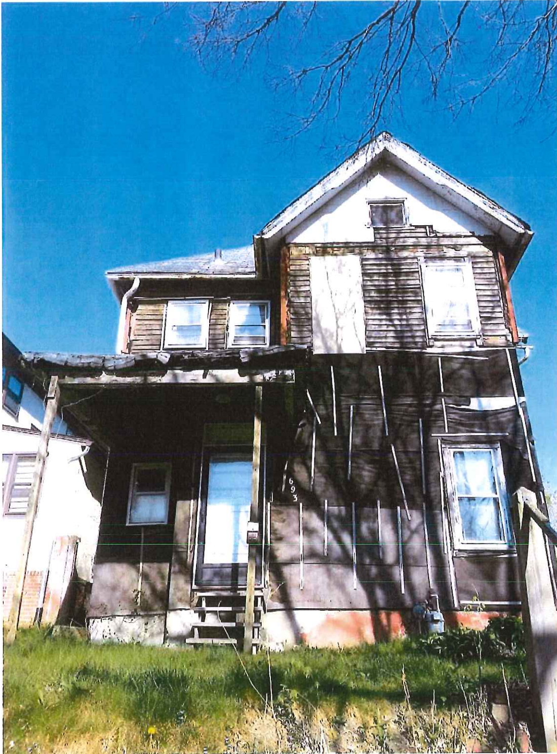
1-W Edward H. Jones House 693 19th St., Des Moines, IA 50314 April 19, 2016 West Elevation
