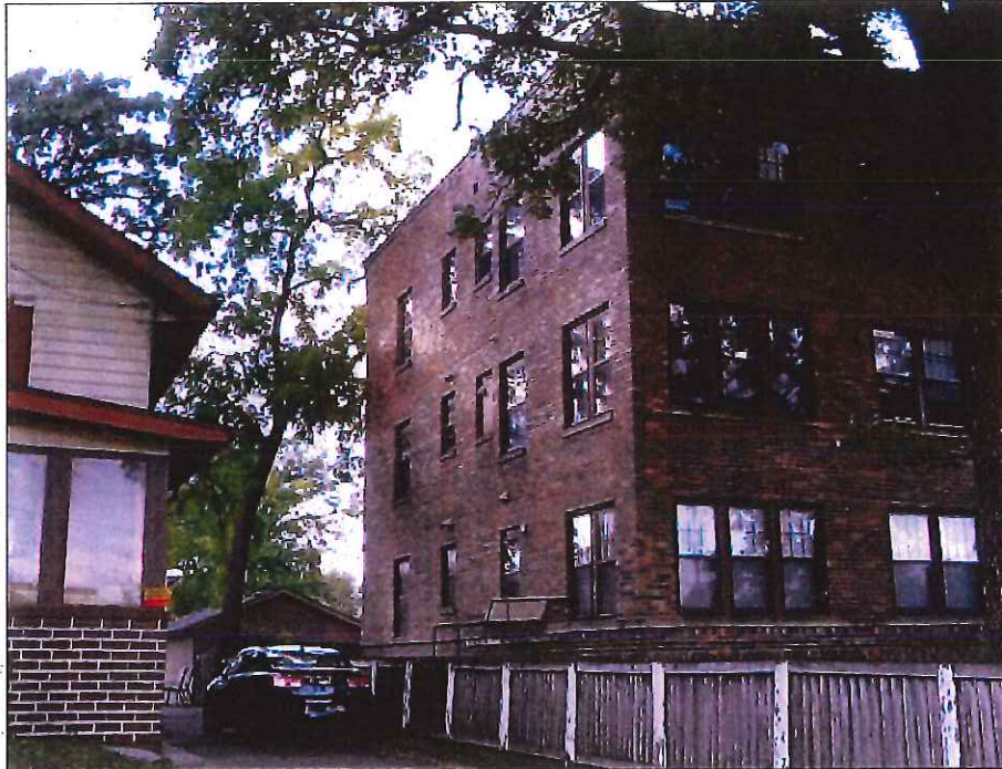
South side of Mirell Flats (77-04888). View to the west-northwest (9/27/17).
