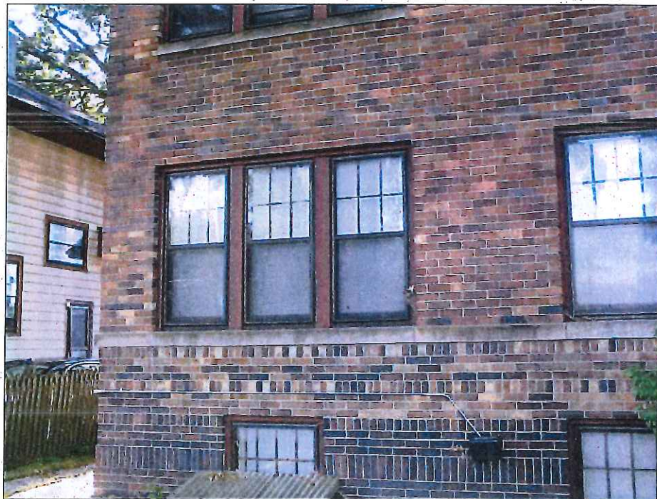
Example of brick courses on east side of Mirell Flats (77-04888). View to the west (9/27/17).
