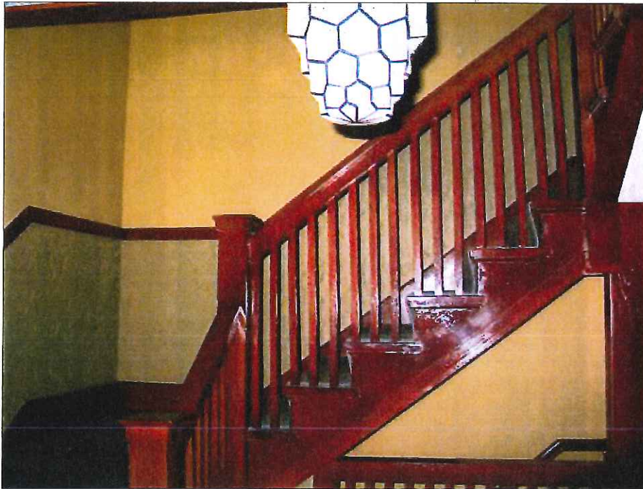
Stairway in Mirell Flats (77-04888). View to the west (9/27/17).
