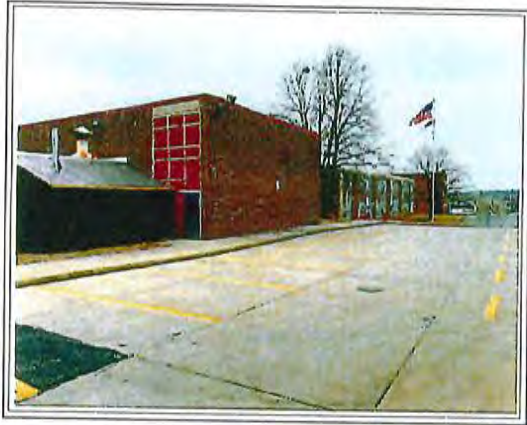
3800 E Douglas Ave Rear View
