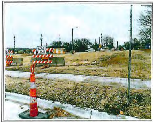
3800 E Douglas Ave E 38th St Closure
