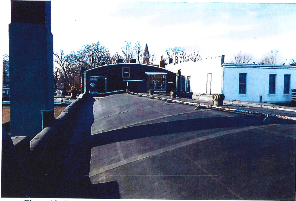
Figure 19: Current roof overview, looking northwest (Jacobsen, 2020)
