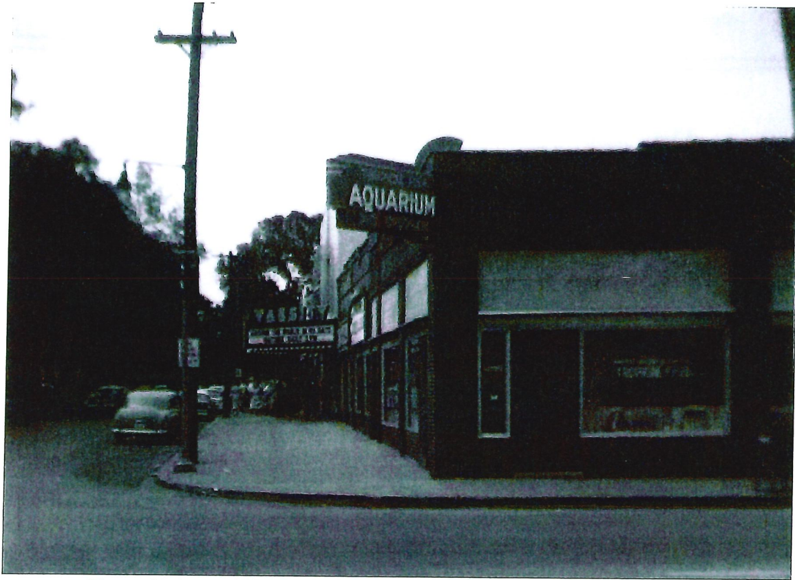
Figure 99: Remodeled marquee and front, looking north, September 1958 (Courtesy of Brian Fridley)
