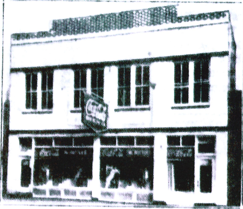
Figure 33: The "New" Coca Cola Bottling Plant, looking east (Des Moines Register, November 3, 1935)
