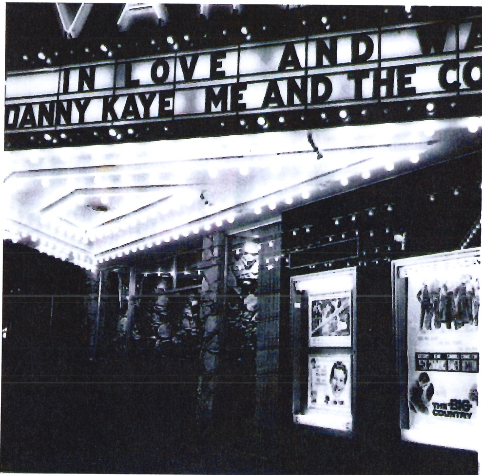
Figure 98: The remodeled façade and marquee, looking southeast and northeast, 1958 (Courtesy of Brian Fridley)
