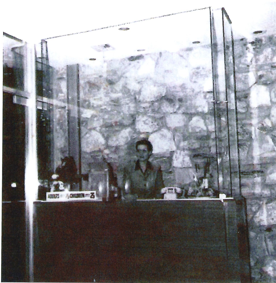
Figure 101: Lobby ticket booth, looking northwest, October 1958 (Courtesy of Brian Fridley)
