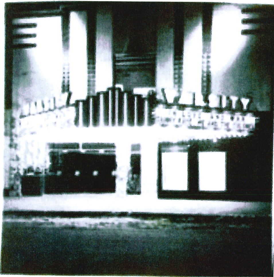
Figure 96: The remodeled façade and marquee, looking northeast, 1958 (Courtesy of Denise Mahon)
