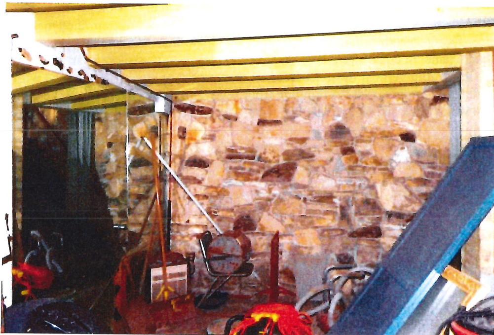
Figure 3: Current basement lobby looking north (Jacobsen, 2020)
