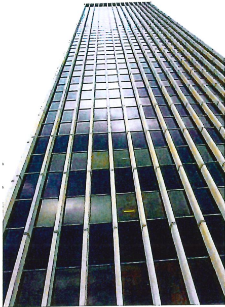
Figures: Left, detail of tower curtain wall bronze tinted glazing and spandrel glass behind vertical mullion fins looking east from rooftop. Right, detail of the canopy entrance into the former Iowa-Des Moines National Bank west wing, with bronze storefront entrances. (Jennifer Irsfeld James, 2020)
