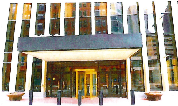
Figures: Left, detail of tower curtain wall bronze tinted glazing and spandrel glass behind vertical mullion fins looking east from rooftop. Right, detail of the canopy entrance into the former Iowa-Des Moines National Bank west wing, with bronze storefront entrances. (Jennifer Irsfeld James, 2020)
