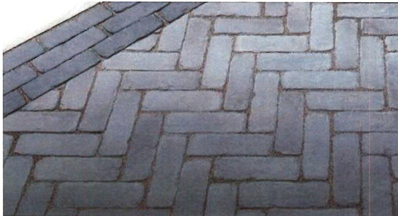
INTEGRAL COLOR PCC SIDEWALK PAVING, SEE DETAIL C501, ADMIXTURE COLOR TO BE SELECTED
