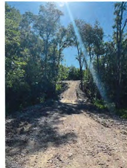
Photo 5: Existing soil stockpile to be utilized as downhill flow trails reuse access road as emergency acces.
