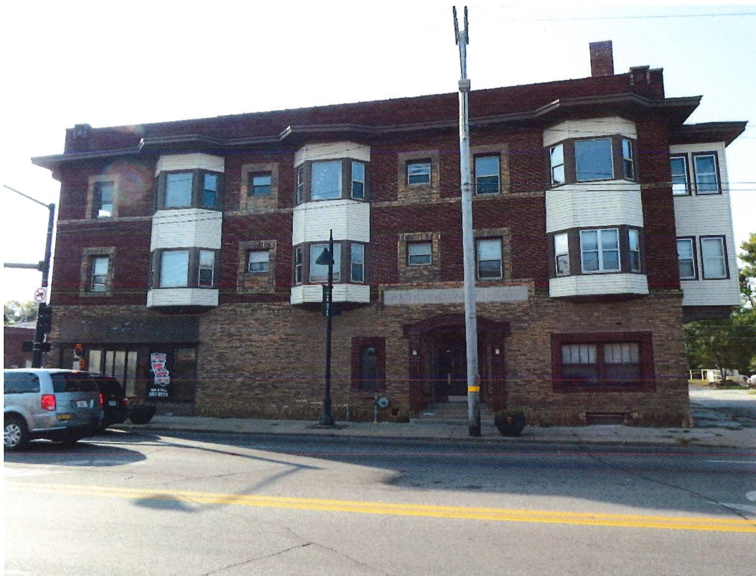
Photo 7: Description: Overview, north facade, looking south
