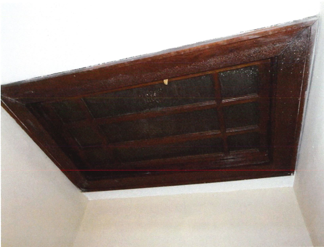
Photo 61: Description: Second floor hall, east end skylight detail, looking northeast
