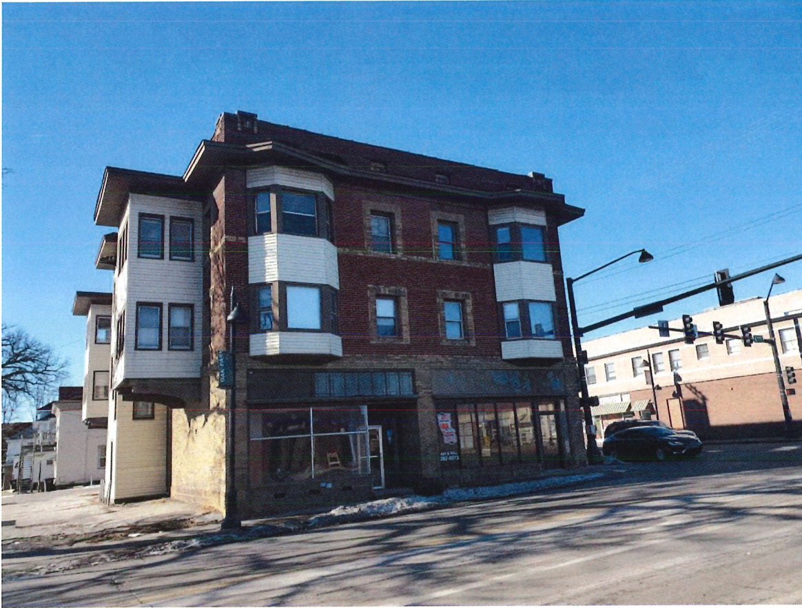
3524 6 th Ave – Eastern Facade
