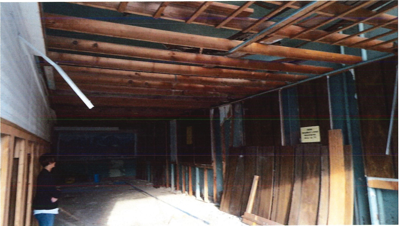
Photo 30: Description: South storefront, looking northwest
