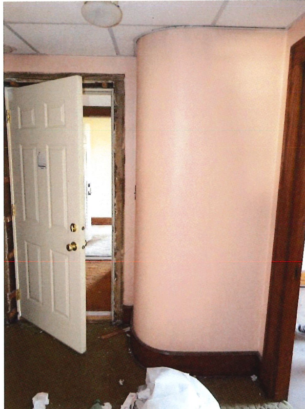
Photo 55: Description: Third floor, apartment 9, entry, curved close wall, looking north
