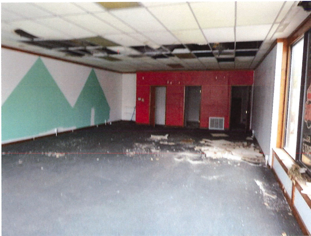
Photo 33: Description: North storefront, looking southwest
