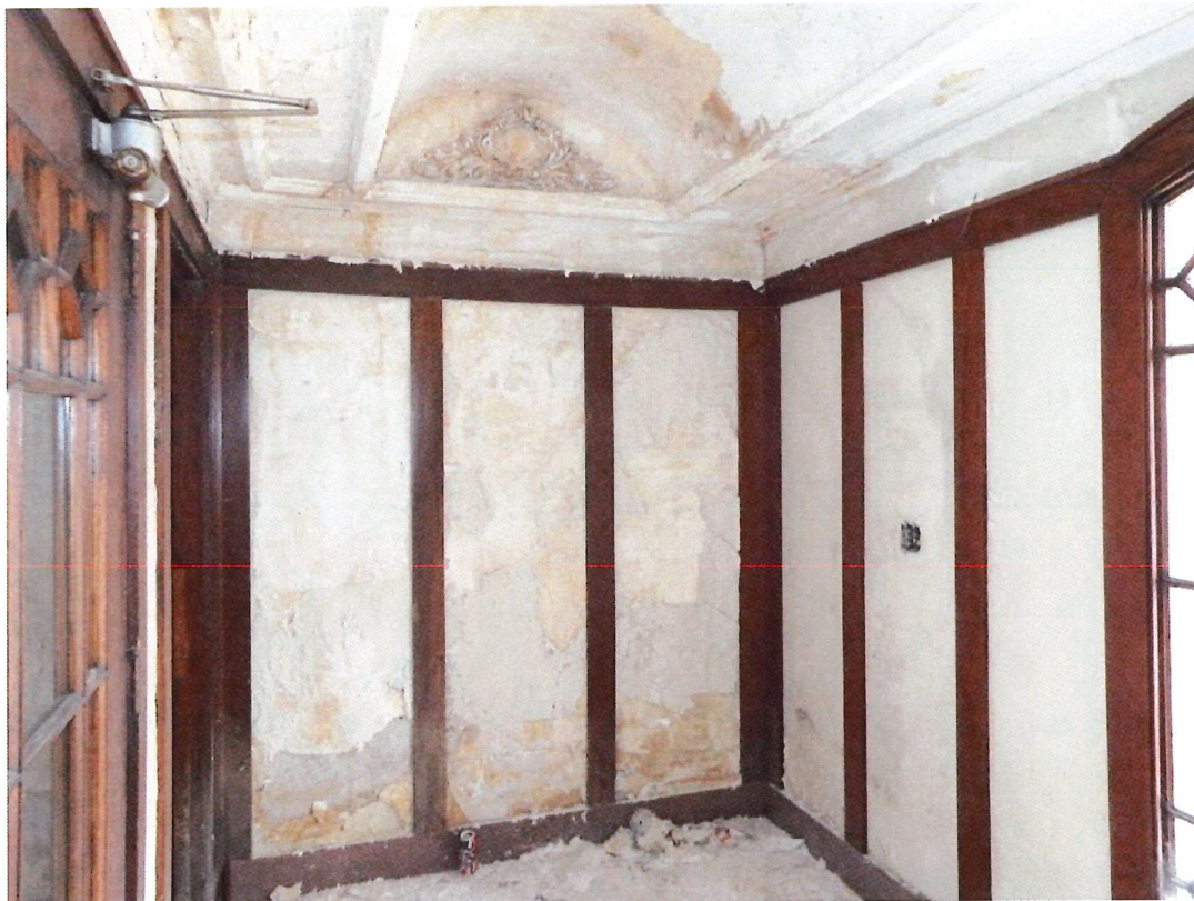
Photo 35: Description: Apartment lobby, looking northwest
