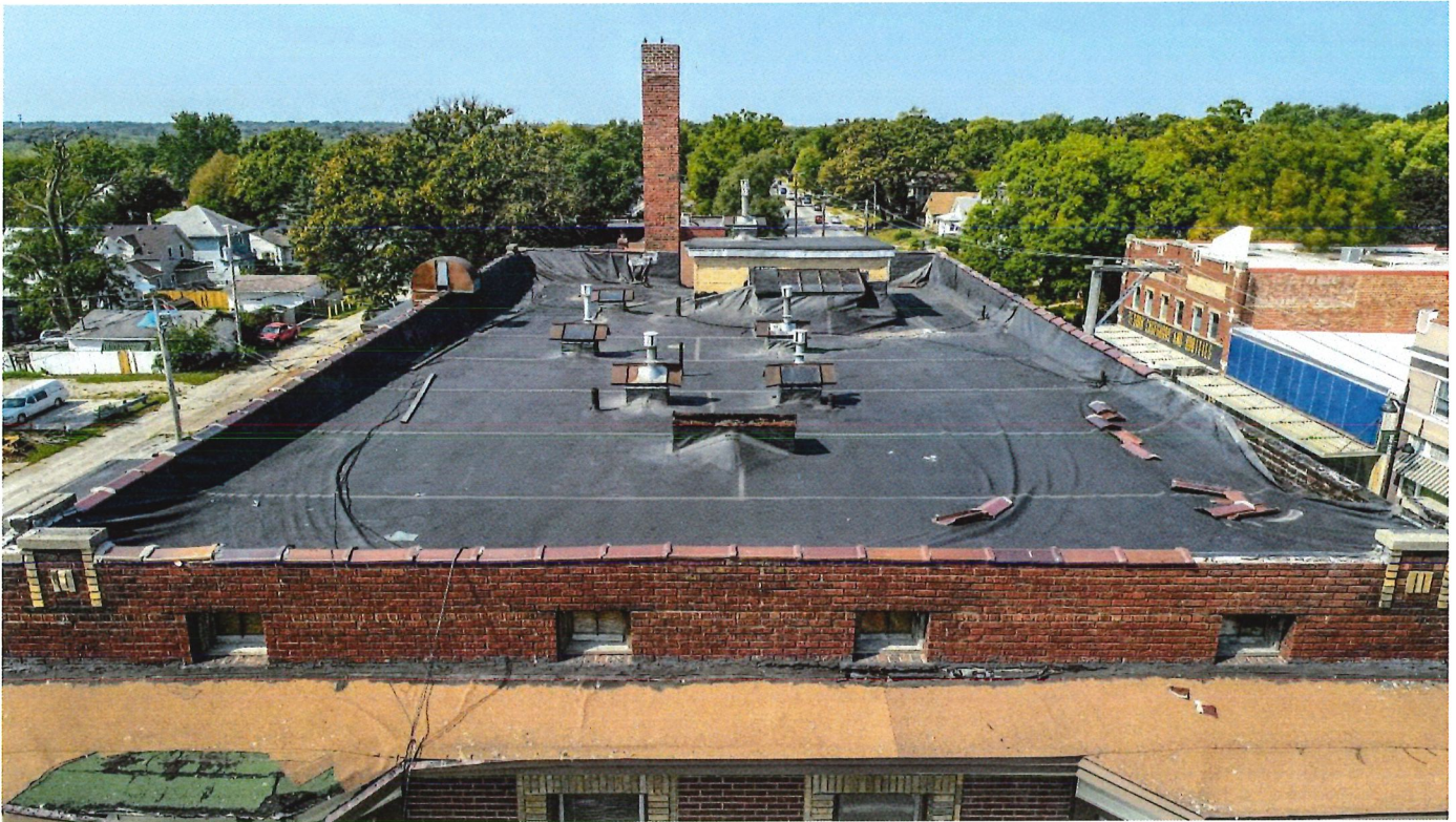
Photo 3: Description: Aerial roof overview, east façade, looking west
