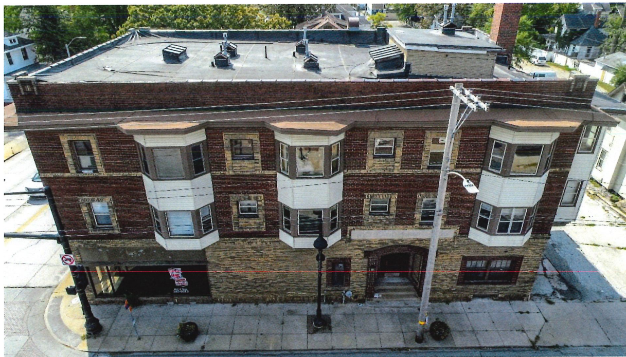
Photo 8: Description: Aerial overview, north façade and roof, looking south
