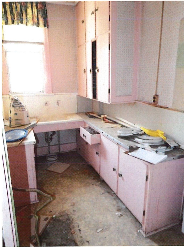
Photo 54: Description: Third floor, apartment 9, kitchen, looking southwest
