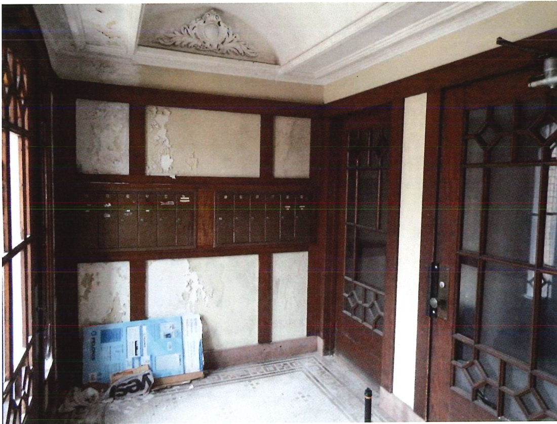
Photo 34: Description: Apartment lobby, looking southeast
