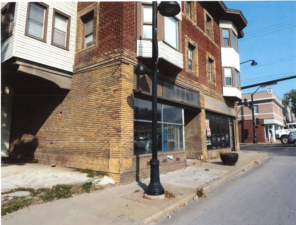
Photo 14: Description: Detail, east façade, looking northwest
