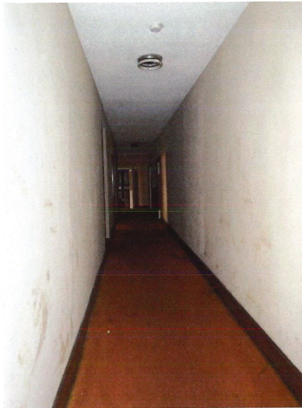
Photo 60: Description: Second floor hall, looking west
