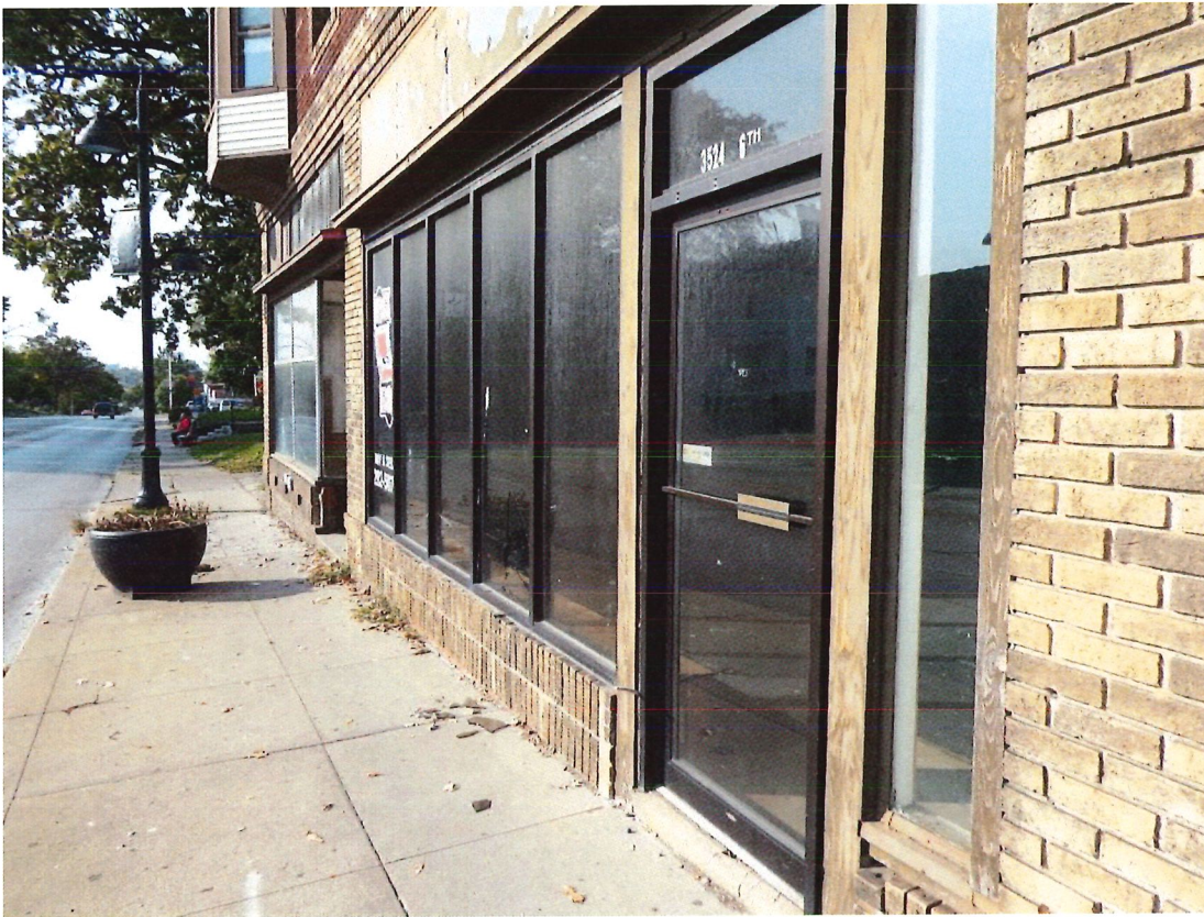
Photo 17: Description: Detail, east façade, storefronts, looking southwest
