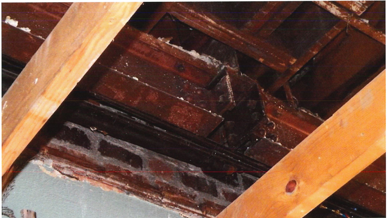
Photo 31: Description: South storefront, steel structural supports along north wall, looking northeast
