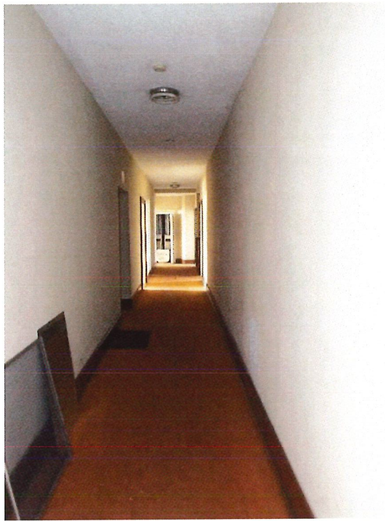
Photo 44: Description: Third floor hall, looking west
