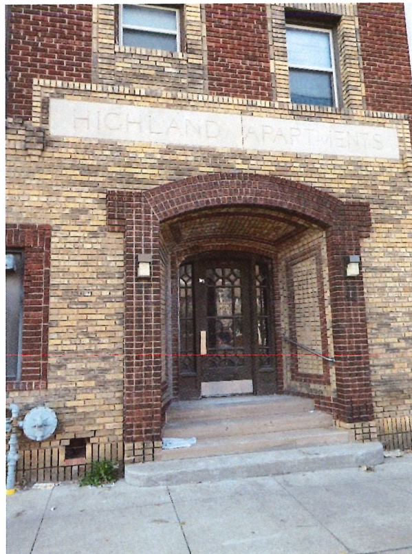
Photo 18: Description: Detail, north façade, apartment entrance, looking southwest
