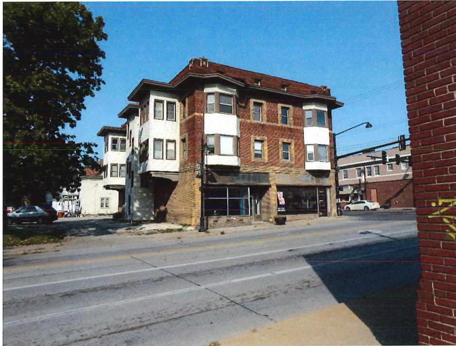
Photo 1: Description: Overview, east façade, looking northwest
