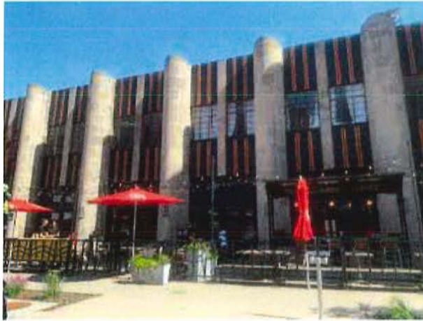
Figure 11. Located at the intersection of Mulberry Street and 9th Street, this building was once a historic fire station at risk for demolition. The City of Des Moines decommissioned this former fire department headquarters with the requirement that the new owner use historic tax credits to rehabilitate the property. After purchase in 2013, the building was renovated and has since housed classes, performances, and a restaurant. 1 The building was listed to the National Register of Historic Places in 2014 as the Des Moines Fire Department Headquarters: Fire Station No. 1 and Shop Building. (Source: KKC)
