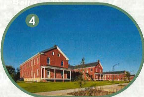
Figure 15. Fort Des Moines (Source: Architect Magazine)
