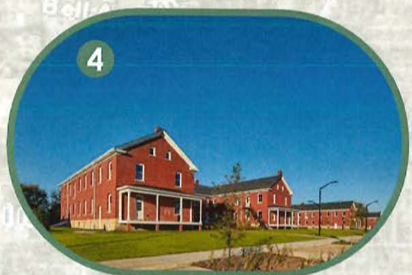
Figure 15. Fort Des Moines (Source: Architect Magazine)
