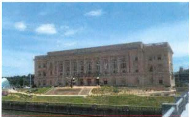
Figure 25. Des Moines City Hall (Source: KKC)
