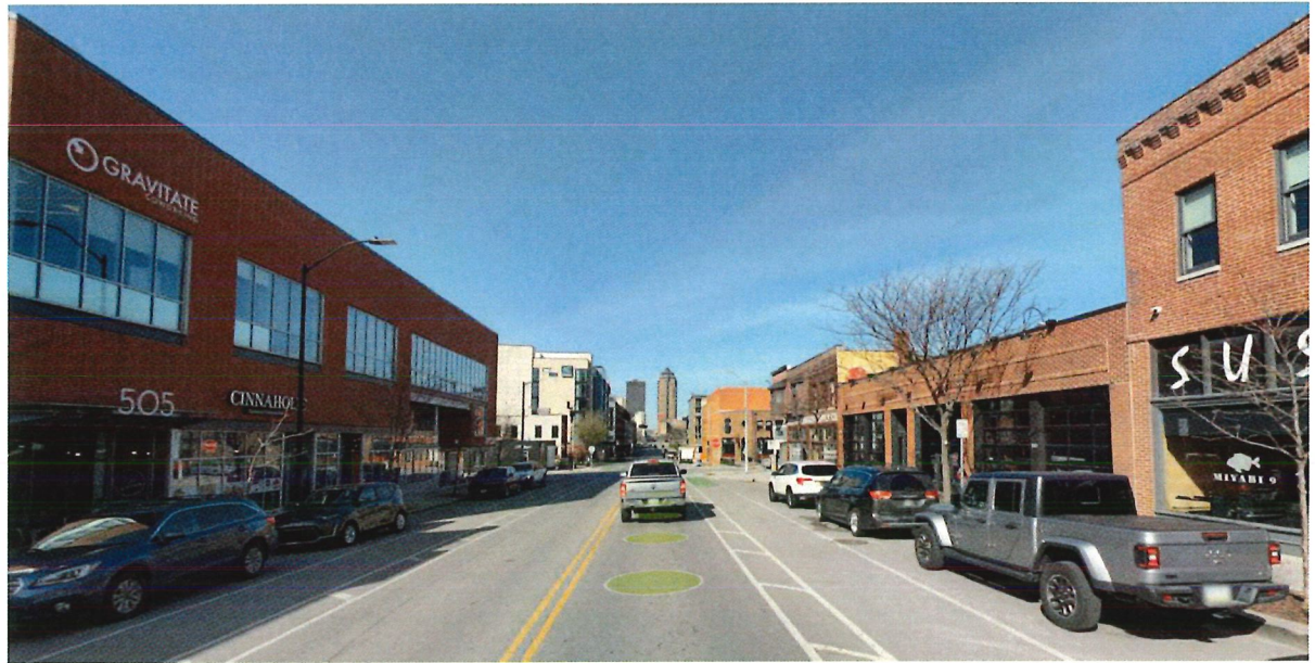
Underground District looking west along the E Grand Ave corridor
