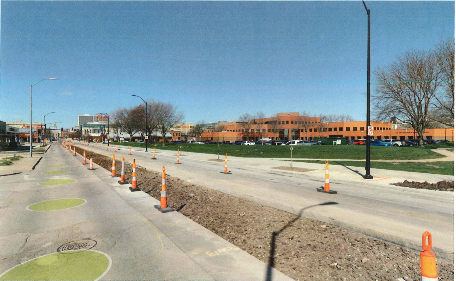
Underground District looking west along the E Court Ave corridor
