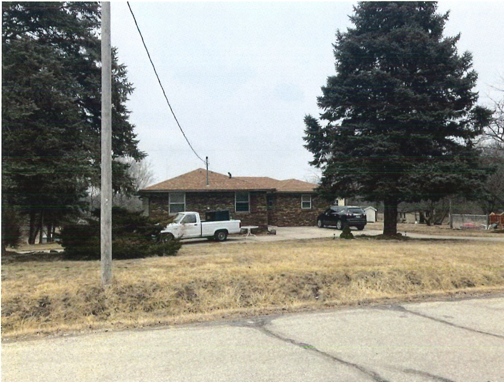
View of the existing one-household residence at 4789 NE 33 rd Court.
