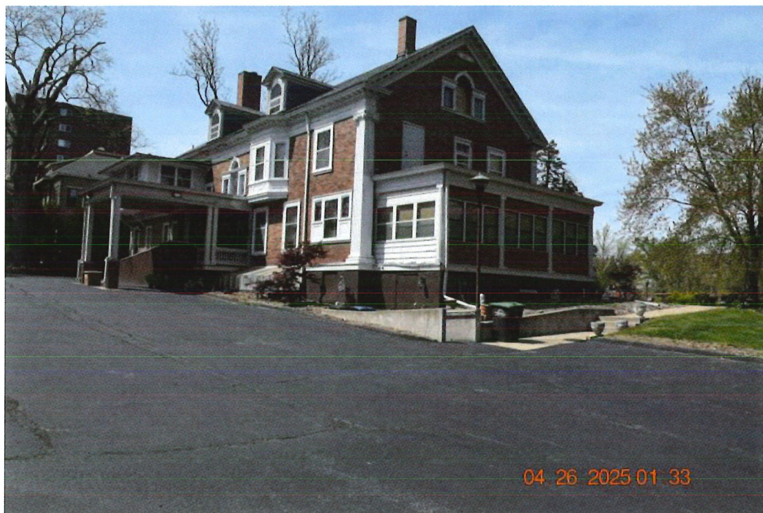
Photo 3: South elevation, looking NW
