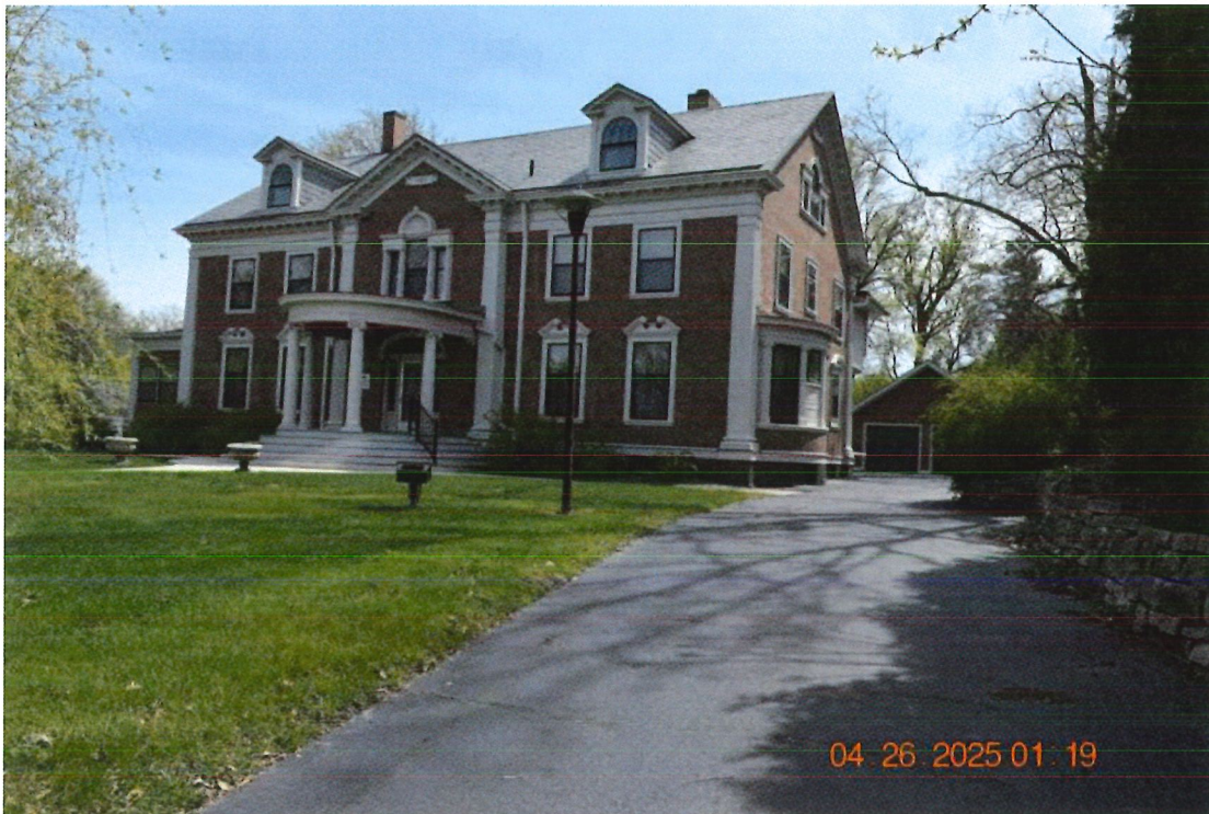
Photo 17: North façade and entry driveway, looking south
