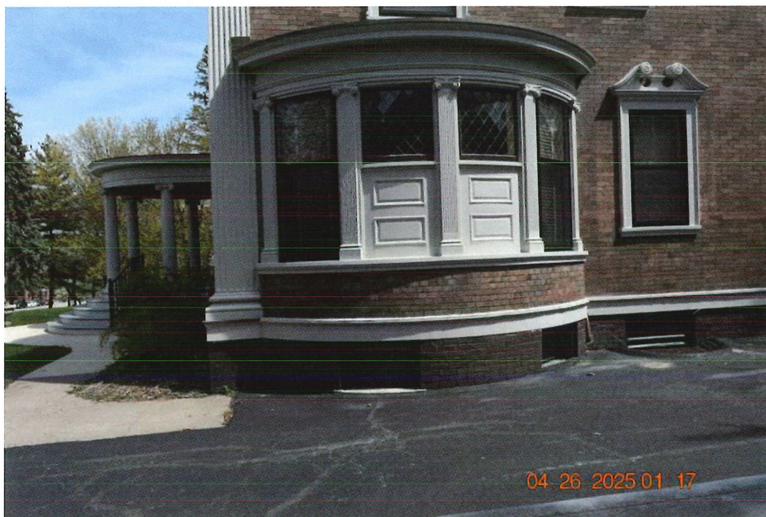
Photo 13: West elevation showing bay window, looking east.
