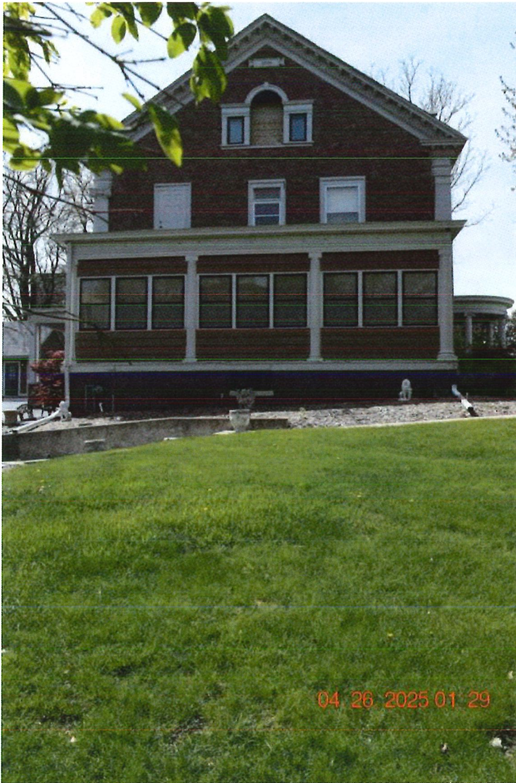
Photo 22: East faced, looking west.
