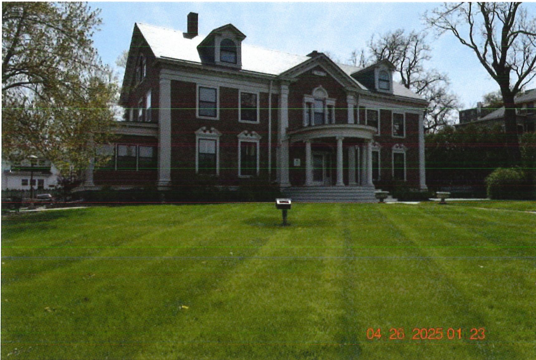
Photo 21: Front facade, looking sw
