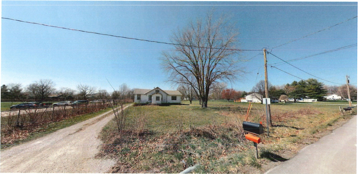
A view of the subject property looking northeast from Northeast 11 th Court.
