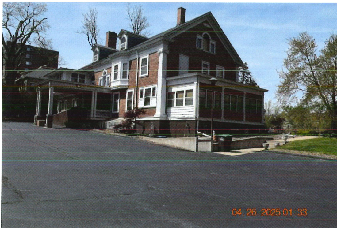
Photo 3: South elevation, looking NW
