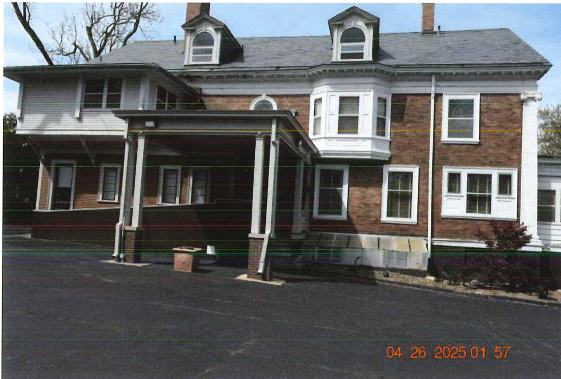
Photo 2: South elevation, looking north
