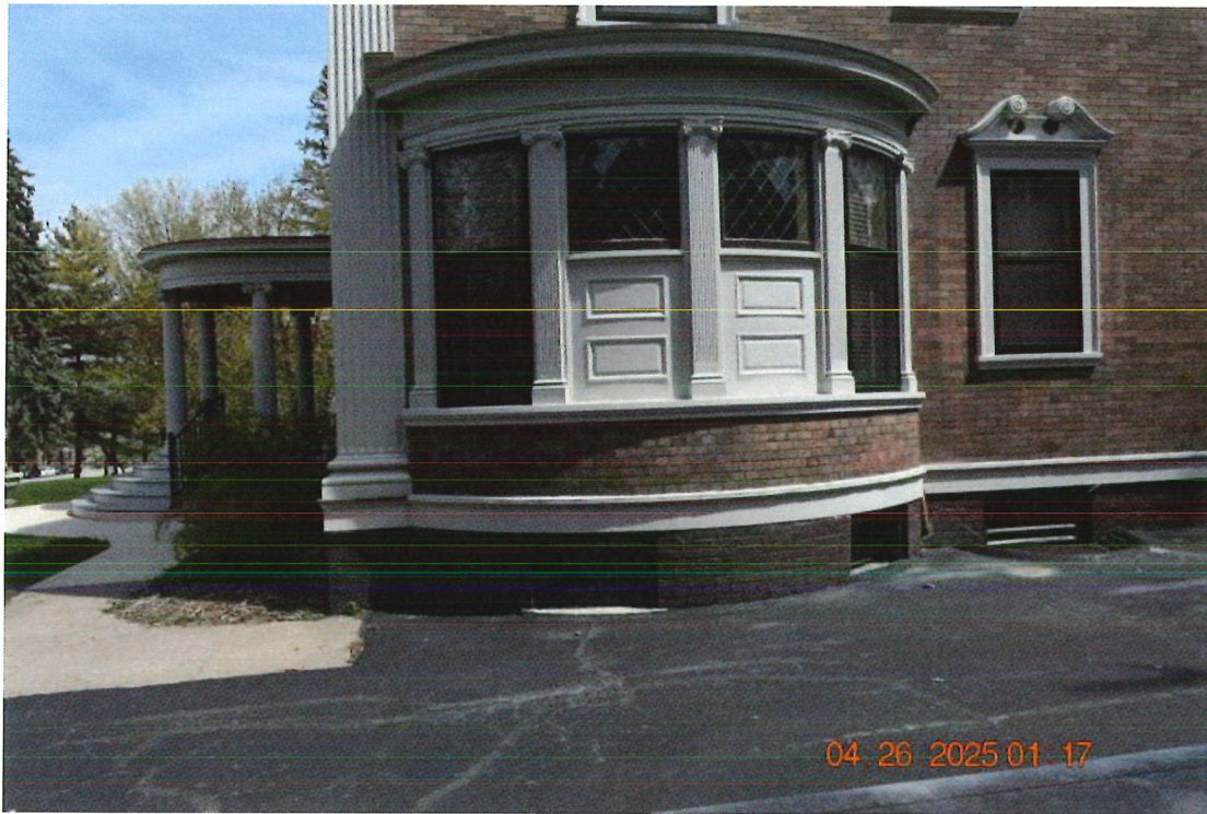
Photo 13: West elevation showing bay window, looking east.
